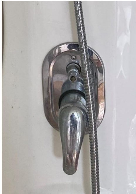
Figure 11 - Temperature control dial missing from shower
