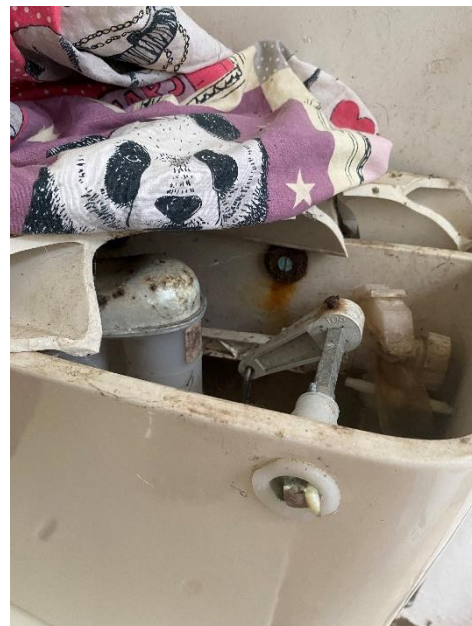
Figure 13 - Flush handle missing from toilet
