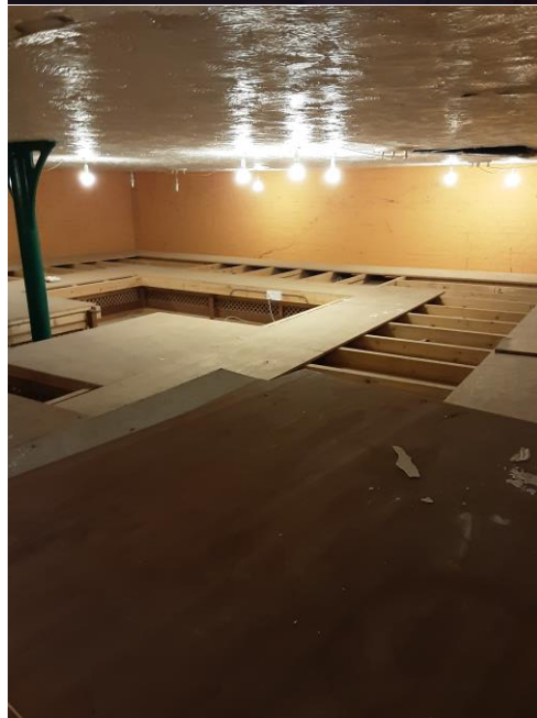
Photograph 6 Void in the Dolls House Museum showing lighting for the display cabinets below.
