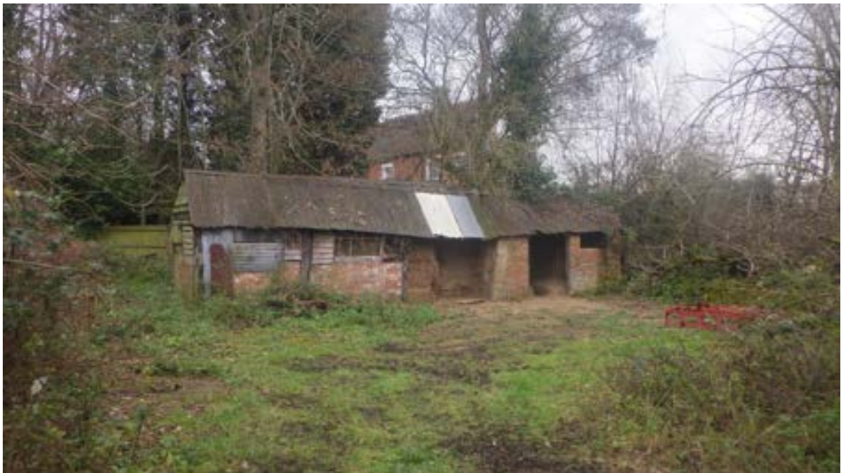
Plate 32: Extant brick building, looking east
