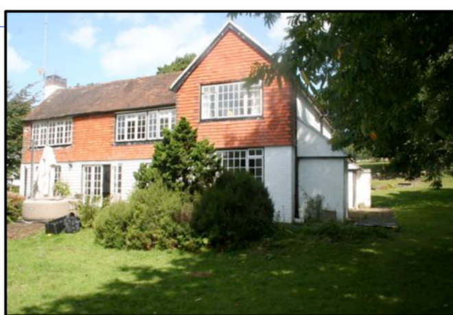
Rear Elevation looking North West
