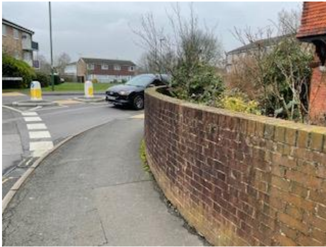
Figure 4: Wall restricting intervisibility at proposed crossing point.
