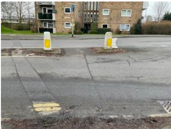
Figure 2: Ponding and detritus at crossing point.
