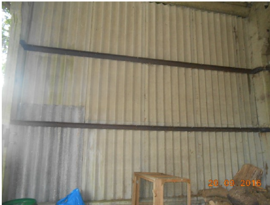
P5 – Internal elevations – RSA sheeting rails
