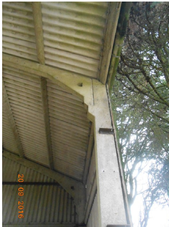
P8 – Typical portal frame post and rafter connection
