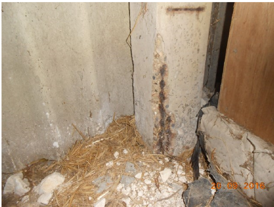
P12 – Local spalling and corrosion to post
