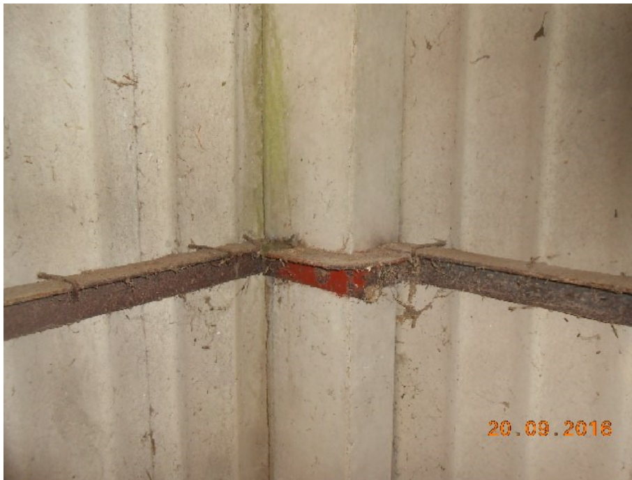
P9 – Steel angle bracket to corner post
