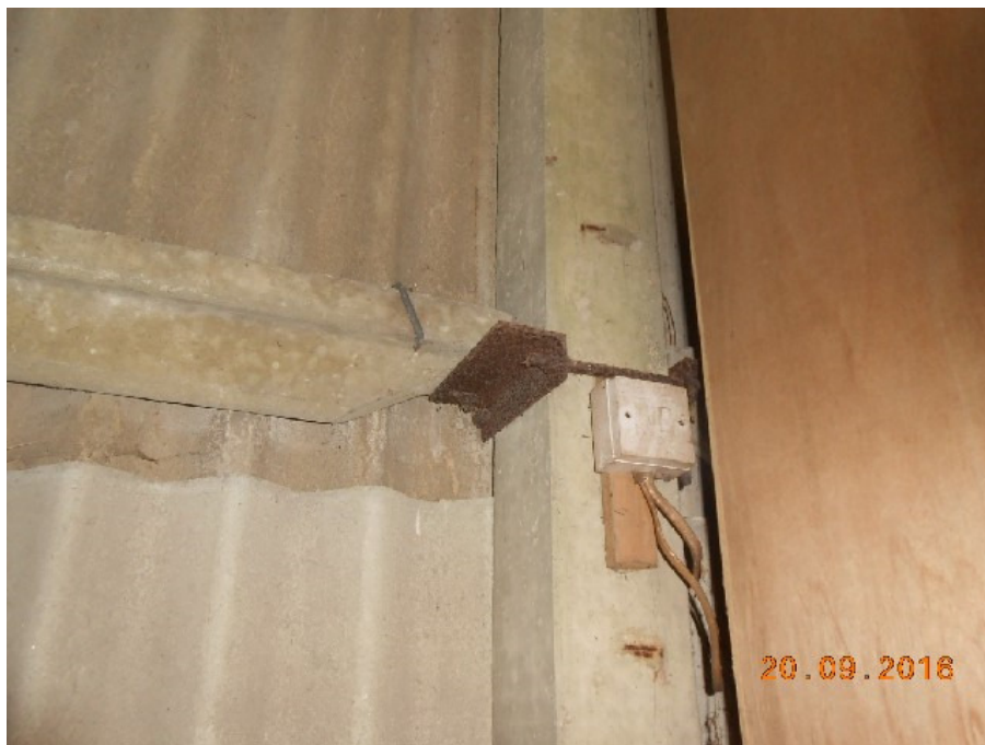
P10 – Steel angle bearing for pre-cast concrete sheeting rail
