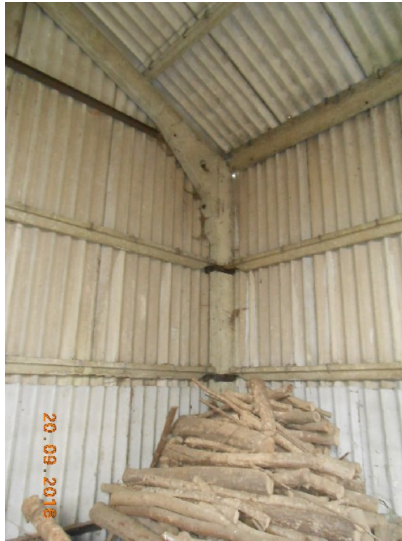
P7 – Corner post with junction of pre-cast concrete sheeting rails
