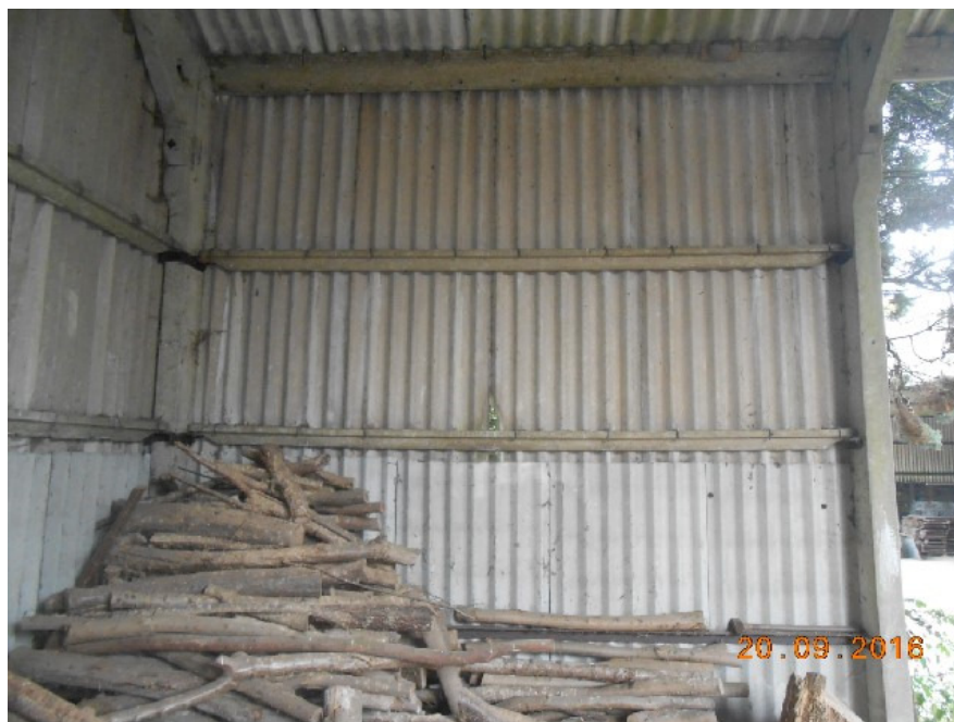
P4 – Internal elevations PCC rails
