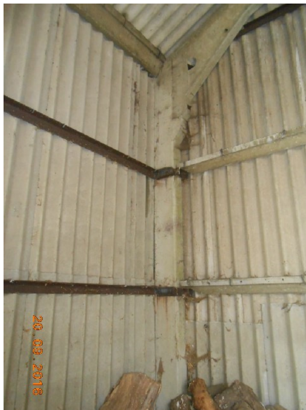
P6 – Corner post with rolled steel angle junction and pre-cast concrete rails
