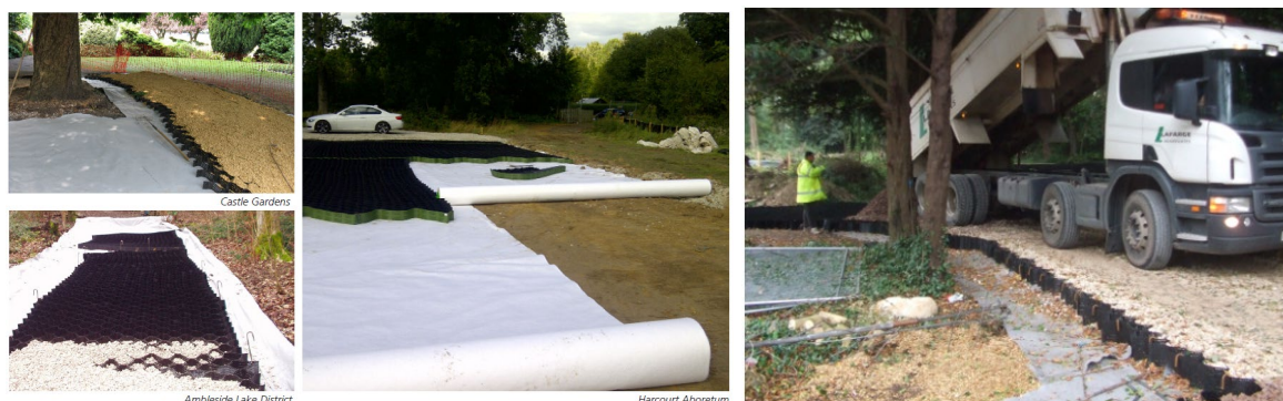
Figure 8: CellWeb® TRP depth variations and applications 7 .
