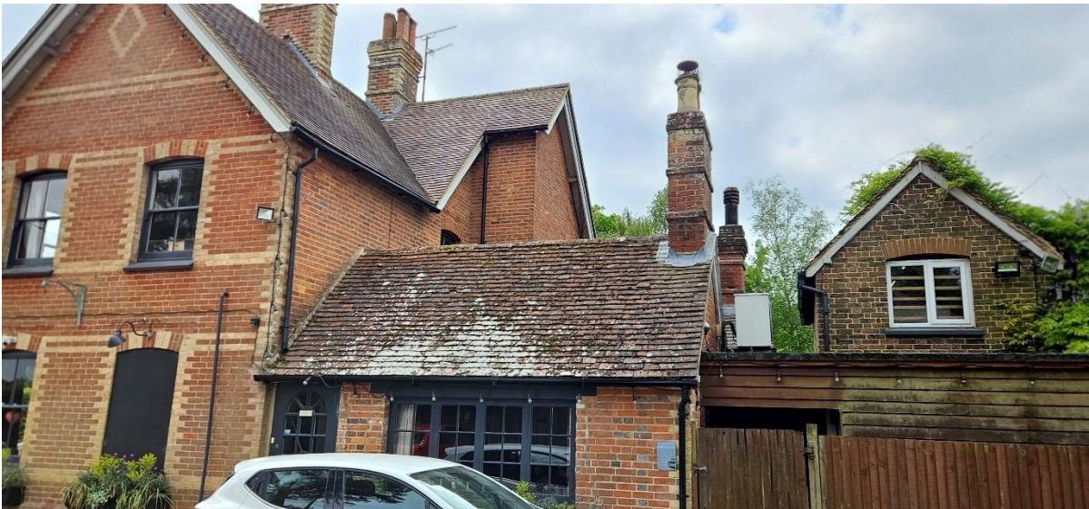
Photo 2 – Roof tiles of the southern aspect. Numerous lifted, displaced or cracked tiles were noted across each roof section.
