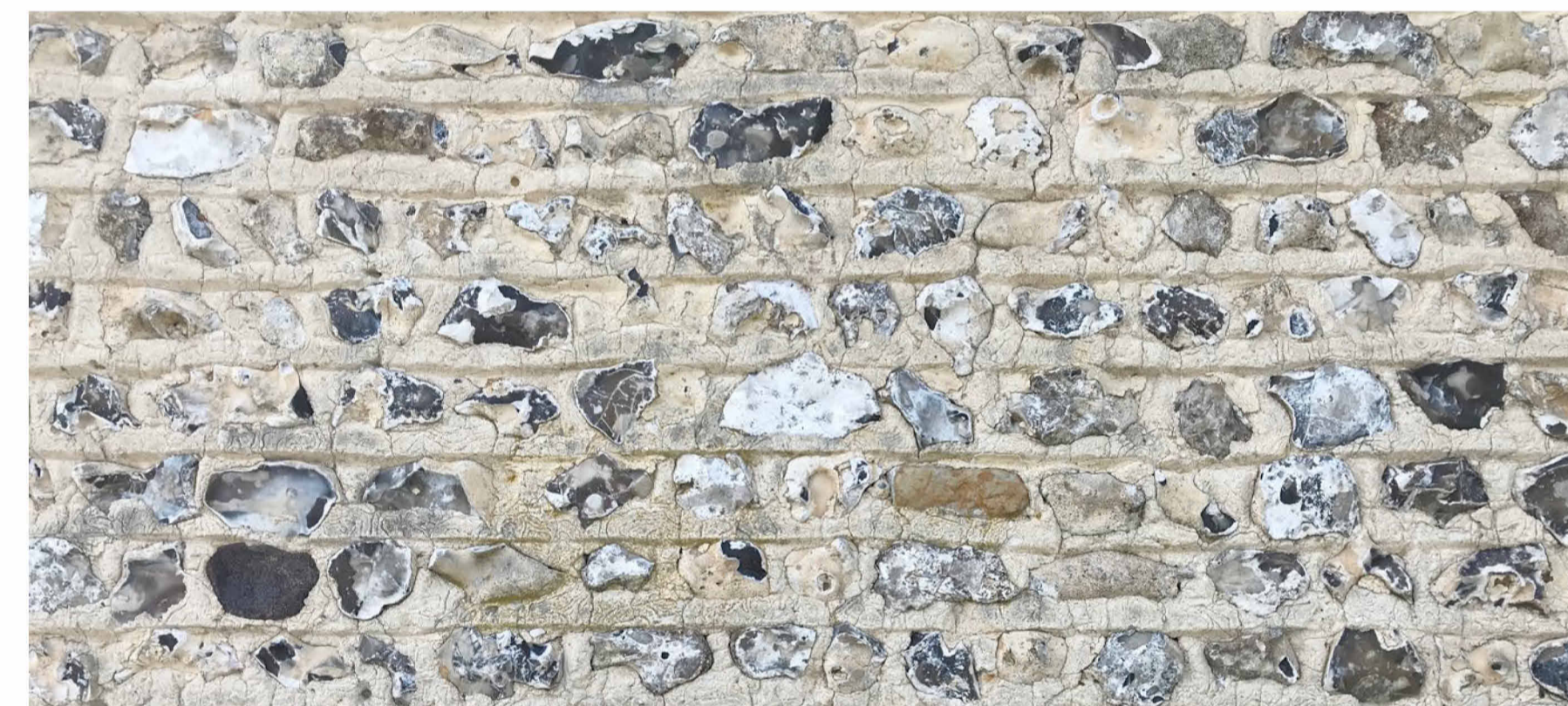
FLINT: Mixed coursed flint block, laid in lime mortar
