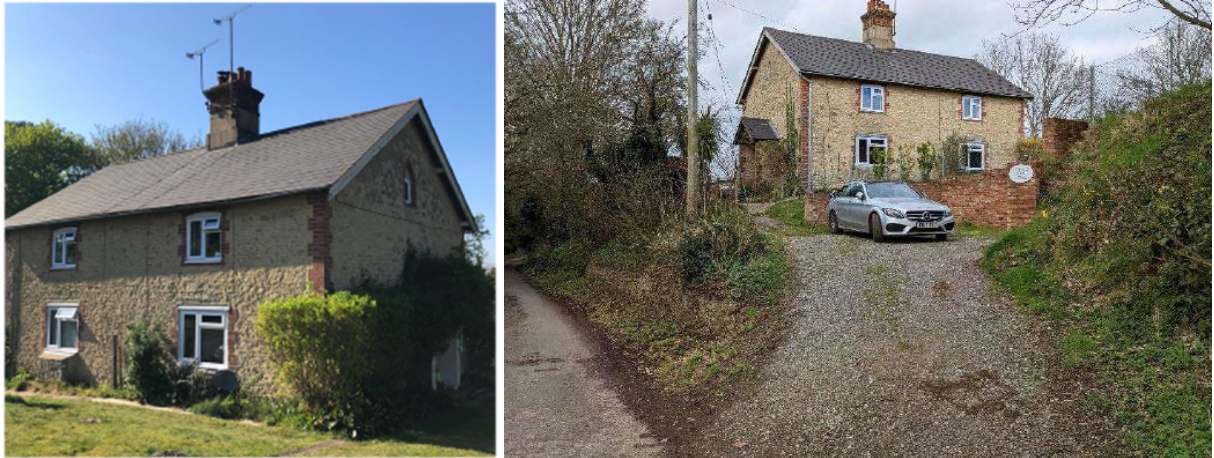
Figure 2.2 - Photograph of No.s 1 and 2 Threals Farm Cottages
