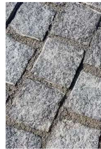
Granite setts (surface transitions)
