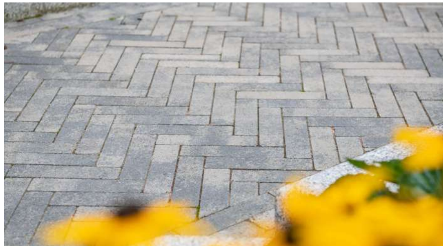
Permeable paving for parking bays
