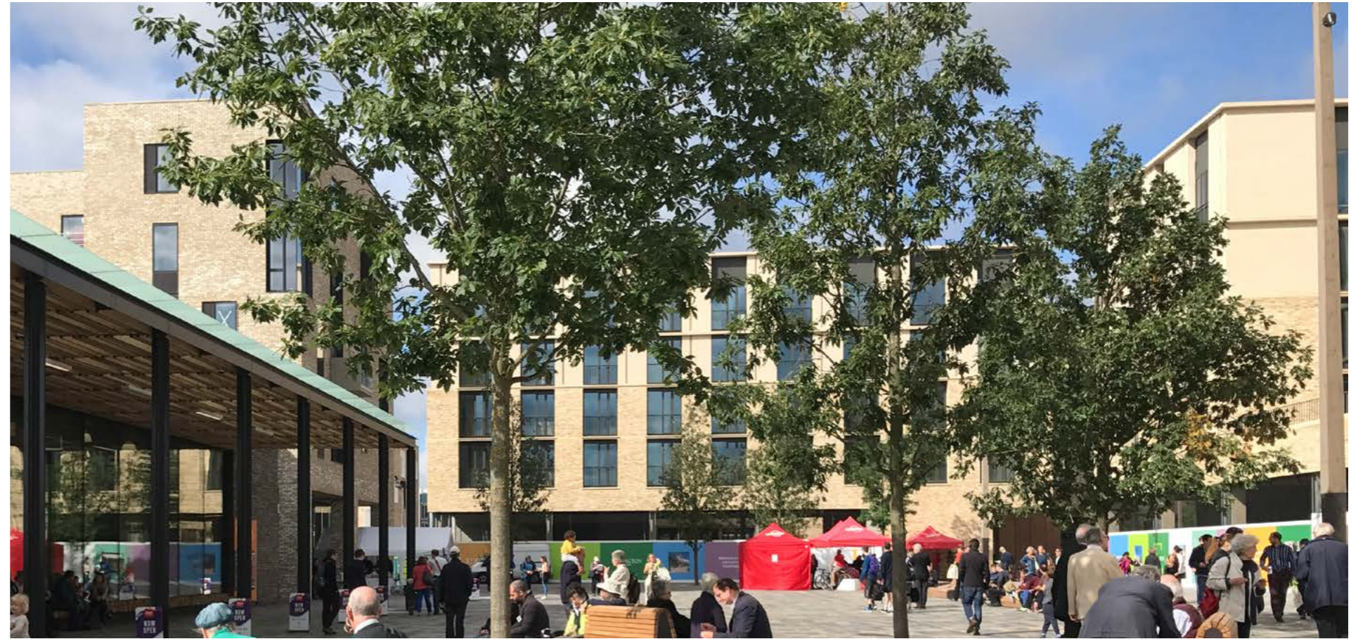
FIGURE 212 Taller building within the local centre
