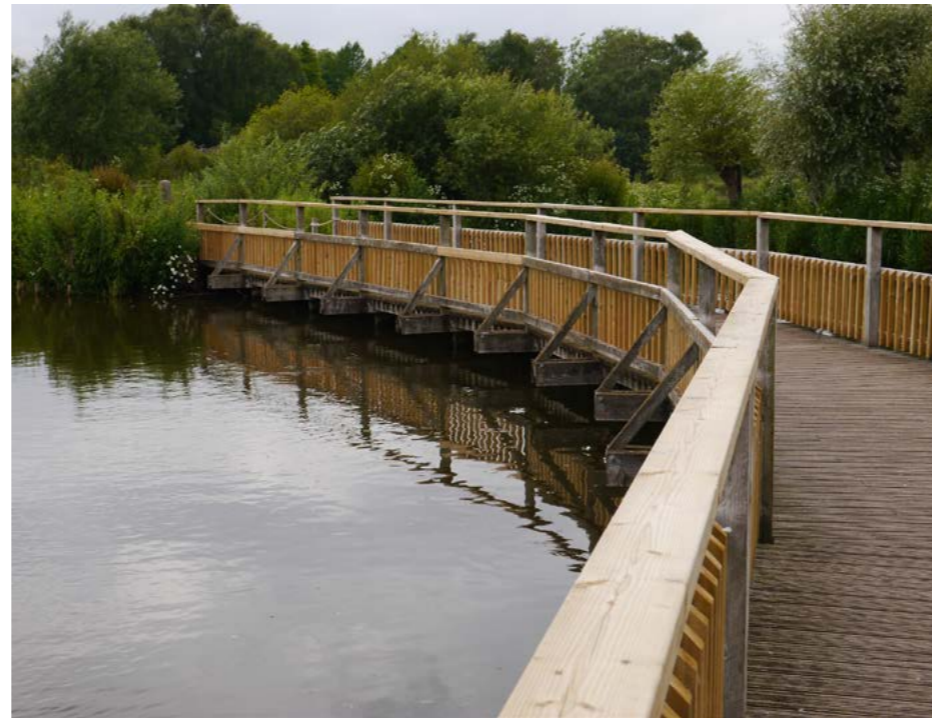
FIGURE 179 A new bridge similar to the above would provide cycle and pedestrian connections across Ifield brook towards Ifield Station
