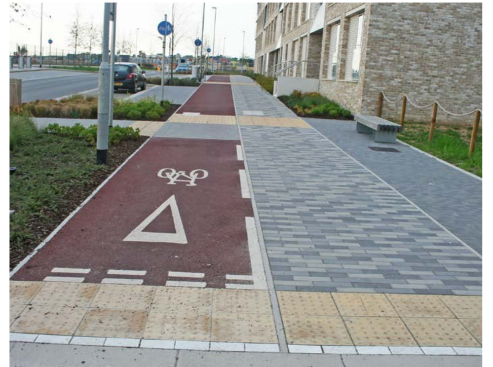
FIGURE 182 On street routes will be separated from the vehicle carriage way planting by green verges and planting. Eddington Cambridge
