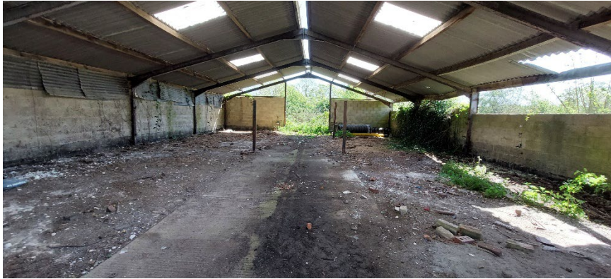
Photograph No: 18 – Internal structure of building B04 looking east, with sky lights and gaps at the eaves visible. Building generally open with no doors present.
