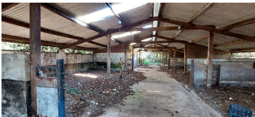
Photograph No: 17 – Internal structure of building B01 with sky lights and gaps at the eaves visible.
