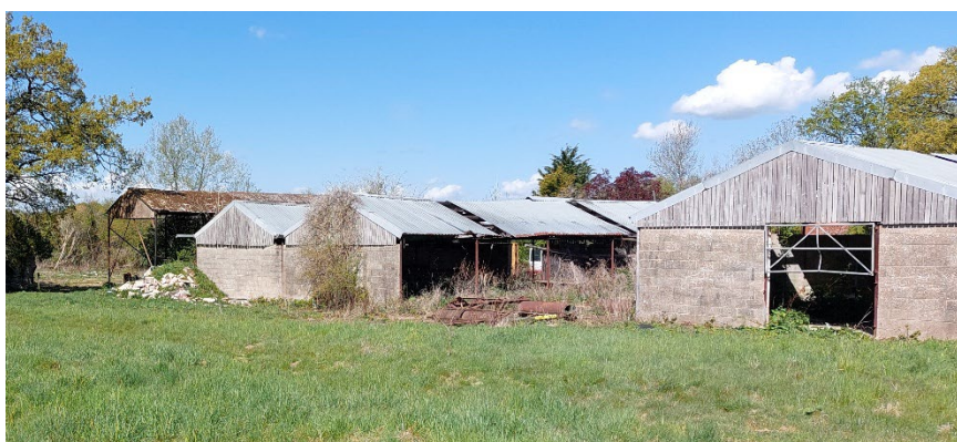
Photograph No: 16 – View across building B02 and B03 with open elevations, gappy roof and lifted ridge sheeting visible.
