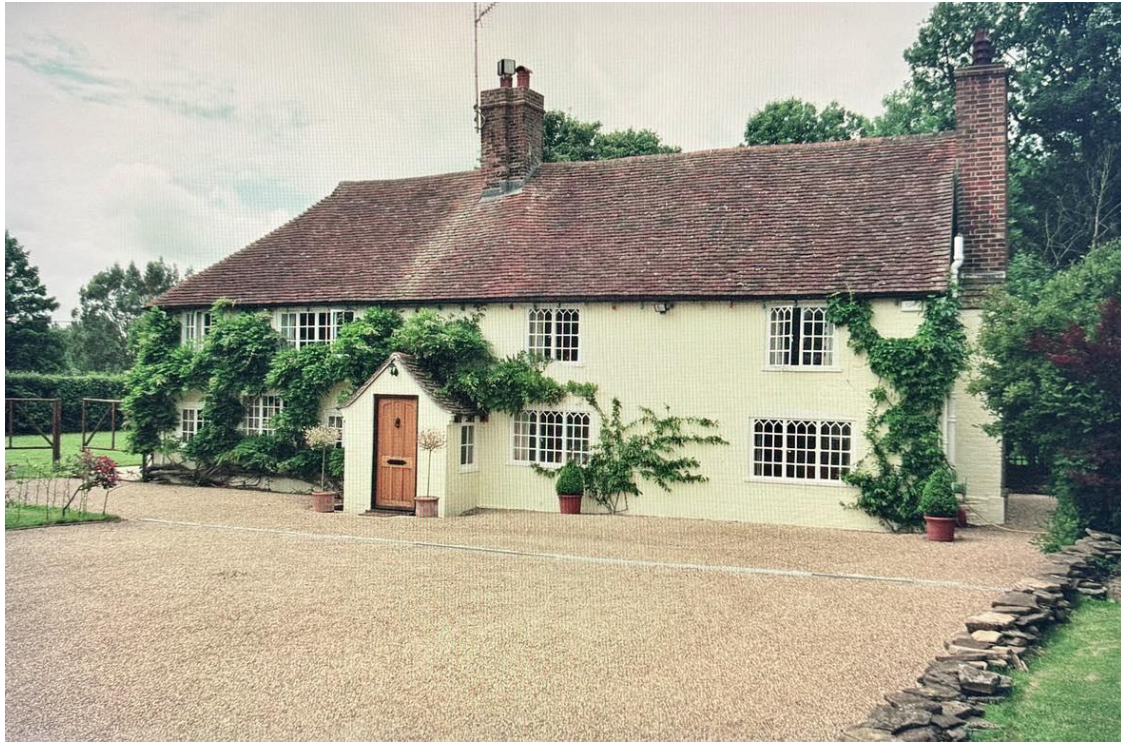
Fig 3: Eastcot dates from the 17 th Century and is a two storey brick built and stone rubble dwelling with a tiled roof. The principal elevation faces east with little to no awareness between it and the proposed site.
