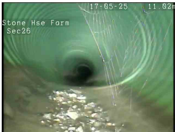
6cd98298-c634-44f6-974c-5e30a6a905c3.png, 00:01:58, 11.20 m Deformed sewer or drain, 15%
