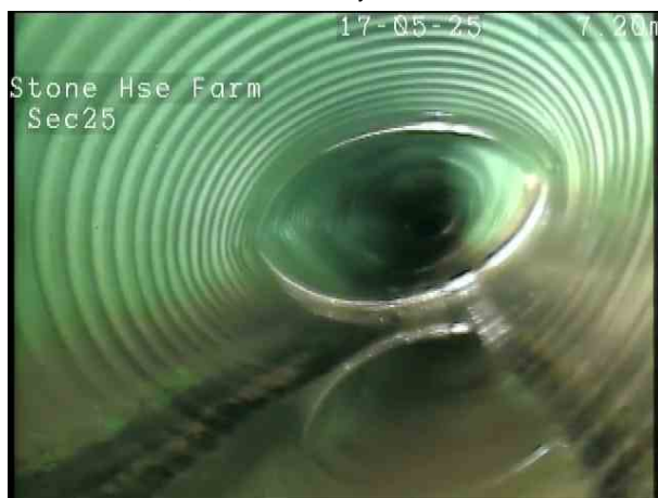
12366aeb-28a8-463f-82ee-57d31161a532.png, 00:00:52, 7.50 m Deformed sewer or drain, 45%
