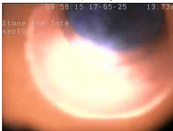
fbbaa57e-3b67-4633-8d7b-8fadf970fa5f.png, 00:00:52, 13.80 m Line deviates up, sharp bend
