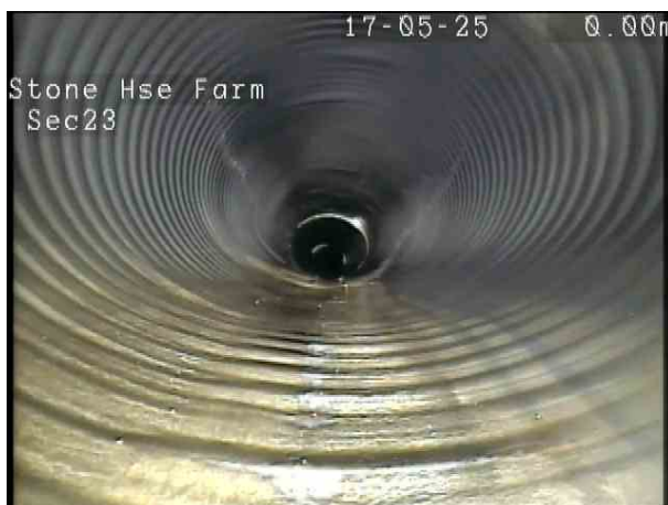
fbf7f5c5-b7f6-4617-a8c5-0d55d098f849.png, 00:00:02, 0.10 m Deformed sewer or drain, 15%
