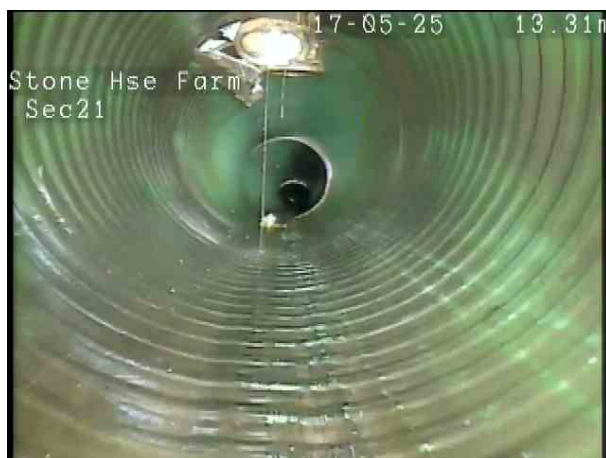
6b0f2f4d-4a35-4beb-a009-e2e8b347bd37.png, 00:01:56, 14.00 m Connection other than junction at 12 o'clock, 100mm dia,
