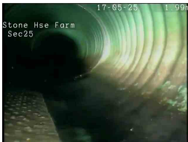
dd64660f-087f-4f2e-873d-646401071db6.png, 00:00:15, 2.00 m Other obstacles, brick or masonry in invert from 5 o'clock to 7
