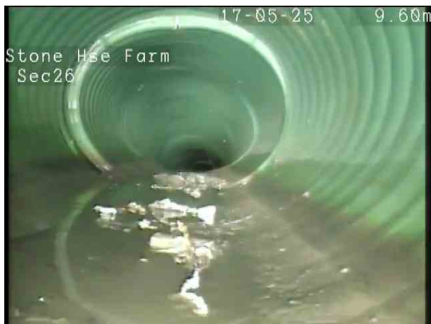
a028aed8-f8fb-4f4c-ab9a-052274501bab.png, 00:01:50, 10.00 m Deformed sewer or drain, 25%
