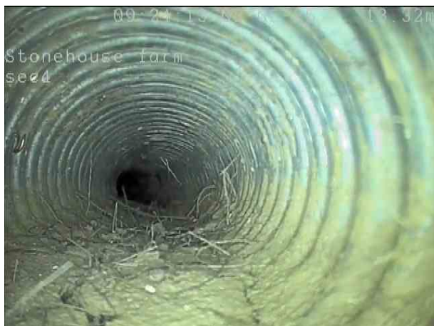
a70a279f-ceb2-420e-978b-bc702a278f05.png, 00:02:38, 13.50 m Settled deposits, fine, 25% cross-sectional area loss
