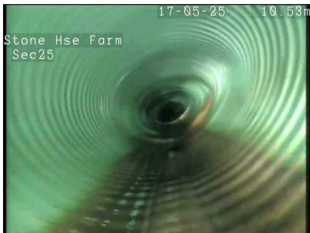
5208e6c7-8ebc-4c5a-82bd-0cd1a3db5e33.png, 00:01:35, 10.60 m Deformed sewer or drain, 30%
