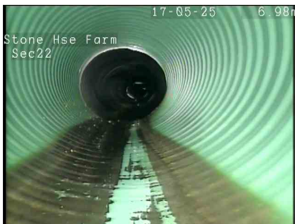
eea8d6d7-b02f-4892-9bdd-4832aadfb6a0.png, 00:00:59, 7.00 m Deformed sewer or drain, 15%
