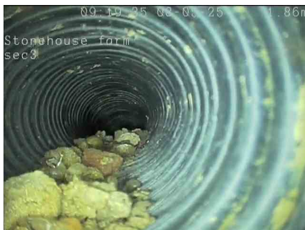
835b38c7-f6be-4f9a-bd41-927da3a1b33a.png, 00:00:13, 1.80 m Settled deposits, hard or compacted, 25% cross-sectional area
