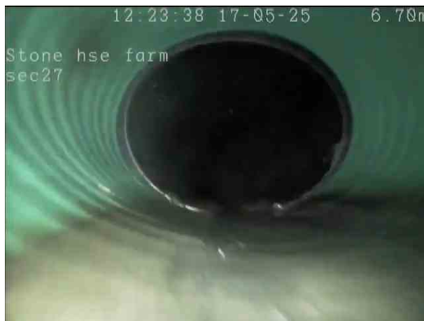
17d22757-c3fd-4c33-910e-5e52593eb4bc.png, 00:00:58, 6.80 m Deformed sewer or drain, 20%
