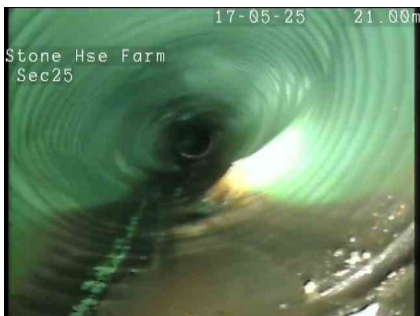
9acab896-a4f8-4573-9648-f059255cb092.png, 00:03:02, 21.00 m Deformed sewer or drain, 45%
