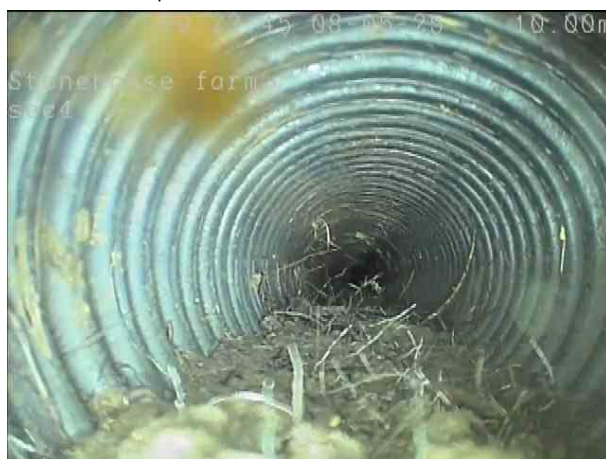
c59c8a99-3d8d-47ac-a172-5cc1ea747f80.png, 00:02:10, 10.00 m Settled deposits, fine, 35% cross-sectional area loss
