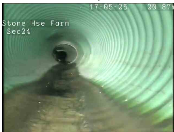
d2c521ea-1e7b-4fda-8963-3a6d69cdd06d.png, 00:02:57, 21.00 m Deformed sewer or drain, 20%
