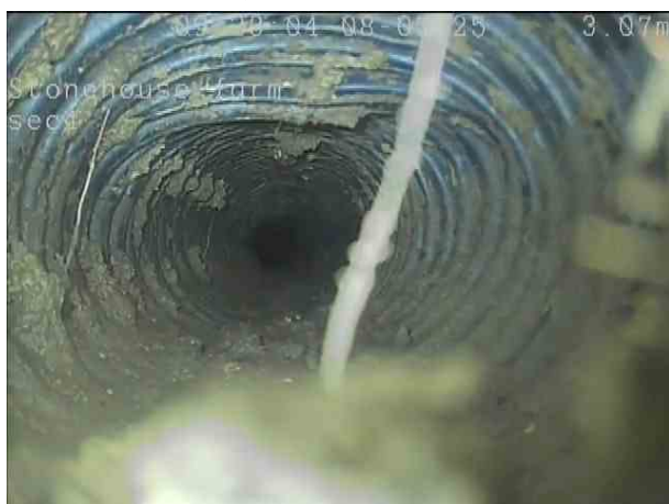
84295523-ce29-40a8-9813-9c39902b9e3a.png, 00:01:29, 3.10 m Deformed sewer or drain, 25%
