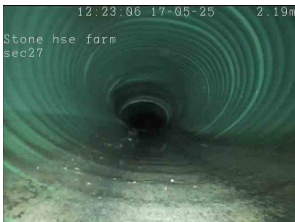
5e369506-e54f-4a0e-86ac-f8af15fd0b05.png, 00:00:26, 2.00 m Deformed sewer or drain, 25%, start
