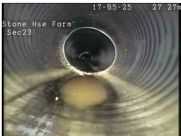
2cb4ab0b-8e54-4902-ab1d-175a7a75332b.png, 00:02:33, 27.50 m Deformed sewer or drain, 15%
