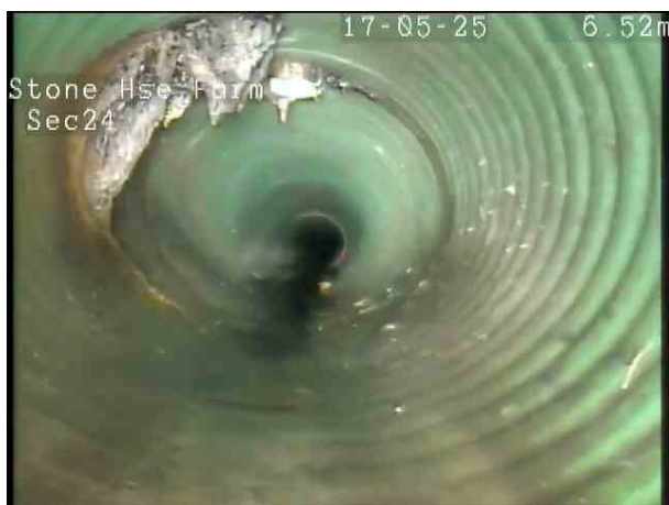
af5239ab-f40b-436a-b478-420914710e4c.png, 00:00:55, 6.70 m Attached deposits, encrustation from 9 o'clock to 12 o'clock,
