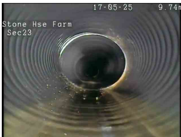
5b24db94-cdf2-4b12-ab19-d851edf7001b.png, 00:01:05, 10.00 m Deformed sewer or drain, 20%
