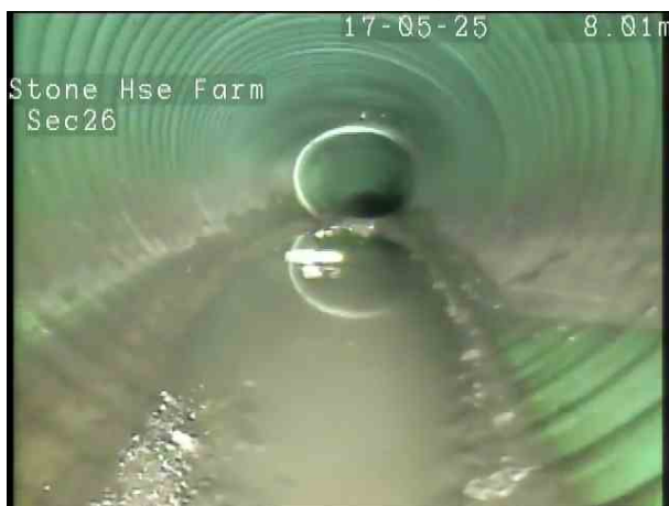
45458732-5374-4e38-8f9a-ae3b790c2857.png, 00:01:33, 8.20 m Water level, 20% of the vertical dimension, deformed
