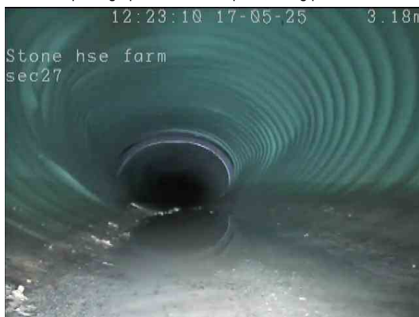
dac68b0f-372b-41bb-8d63-348e5d606ae2.png, 00:00:30, 3.40 m Deformed sewer or drain, 40%
