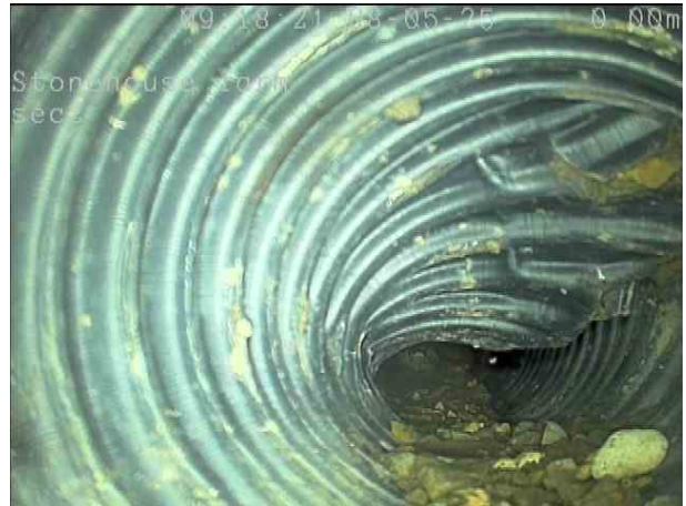
b15bddbd-8303-4808-901c-9ff6eea155cc.png, 00:00:05, 0.30 m Deformed sewer or drain, 70%
