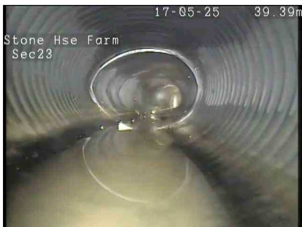
52e5663c-8b45-498f-8a3a-b57c8d704160.png, 00:03:56, 39.50 m Deformed sewer or drain, 35%
