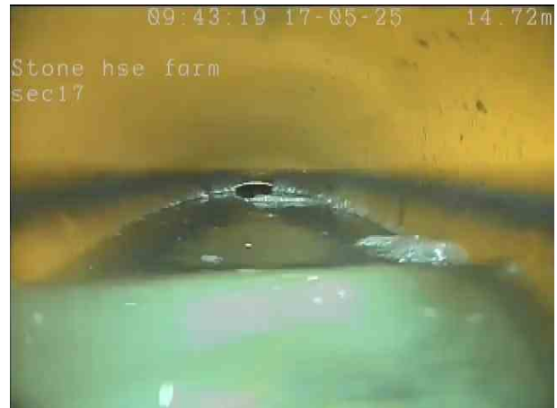
42115dcf-fabe-4b09-add5-df4ee6eef327.png, 00:01:27, 14.80 m Water level, 85% of the vertical dimension, dropped section
