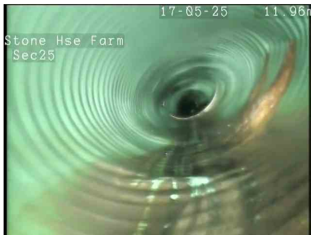
90b14cb1-66c2-43e0-a8da-f199a710dca0.png, 00:01:44, 12.00 m Hole in drain or sewer from 2 o'clock to 4 o'clock
