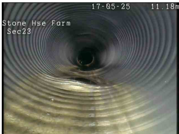
43ddd2e0-a573-4baf-a491-13f54fb589dd.png, 00:01:16, 11.30 m Hole in drain or sewer from 6 o'clock to 7 o'clock
