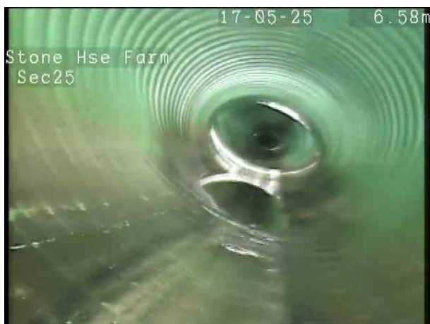
e2952436-e7fe-4fb8-a047-da69afa21ad5.png, 00:00:39, 6.80 m Deformed sewer or drain, 40%
