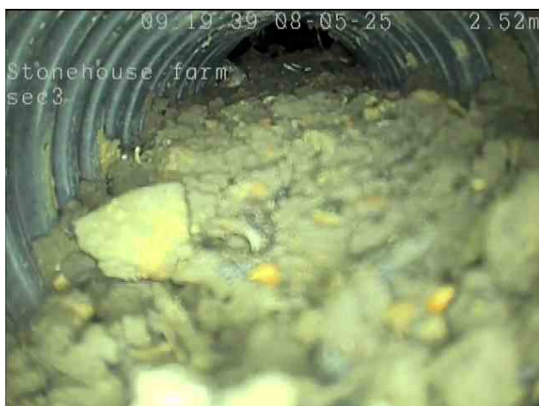
6d72067e-e336-47ff-b0fc-3b5edaefdc7d.png, 00:00:18, 2.50 m Settled deposits, hard or compacted, 85% cross-sectional area
