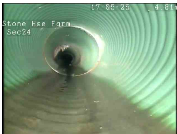
b11ae014-a296-4f4f-9917-cff9ea64299f.png, 00:00:40, 4.80 m Deformed sewer or drain, 10%
