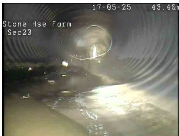
5297a643-8e92-4c66-ab70-4f1185e48459.png, 00:04:28, 43.50 m Deformed sewer or drain, 20%
