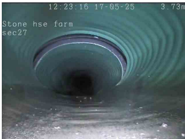
2c299aab-02dc-4b73-bbe7-51f12b5068d1.png, 00:00:36, 4.00 m Deformed sewer or drain, 45%
