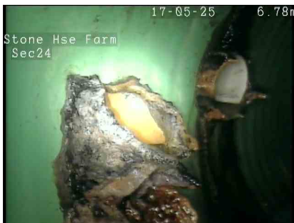
4b4f561f-f90c-4427-90e9-f38d68e4a95f.png, 00:01:16, 6.80 m Connection other than junction at 11 o'clock, 100mm dia, intruding
