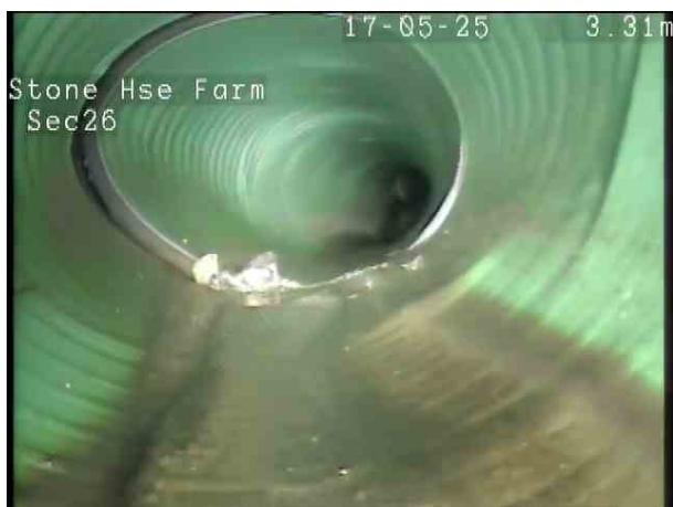
a231dc10-c2ea-4197-96e3-88745ee8fcb7.png, 00:00:41, 4.00 m Deformed sewer or drain, 40%
