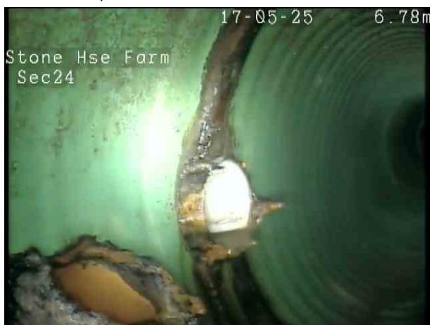
d72e2463-6f0c-4ea1-b976-af6e6ac516d5.png, 00:01:19, 6.90 m Connection other than junction at 12 o'clock, 100mm dia,
