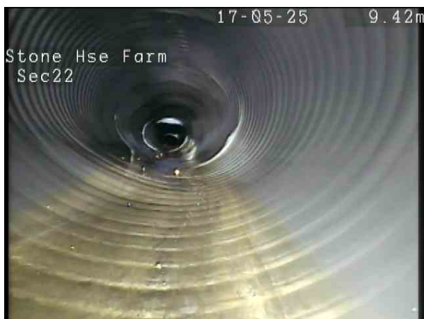
ed06c945-a483-4a6f-bd7e-62f09e7b2bab.png, 00:01:34, 9.50 m Deformed sewer or drain, 20%
