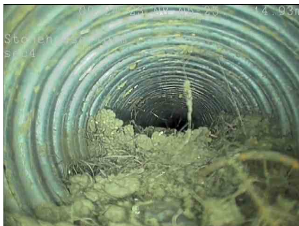
f64ad6e1-52d5-4d0f-800e-38beb7f7f107.png, 00:02:48, 15.00 m Settled deposits, fine, 75% cross-sectional area loss
