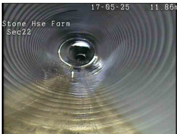
ef924ca4-76c6-45d9-895b-ad59cc0ce47b.png, 00:02:11, 11.50 m Deformed sewer or drain, 25%
