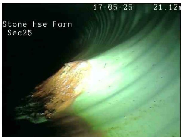
591e2157-abcd-4207-99b0-770ad446df99.png, 00:03:36, 21.20 m Hole in drain or sewer from 4 o'clock to 6 o'clock
