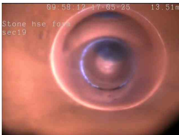
15c02a60-6b0a-4327-ba76-0f79e9b81eef.png, 00:00:49, 13.60 m Junction at 12 o'clock, 100mm dia, serves rwp
