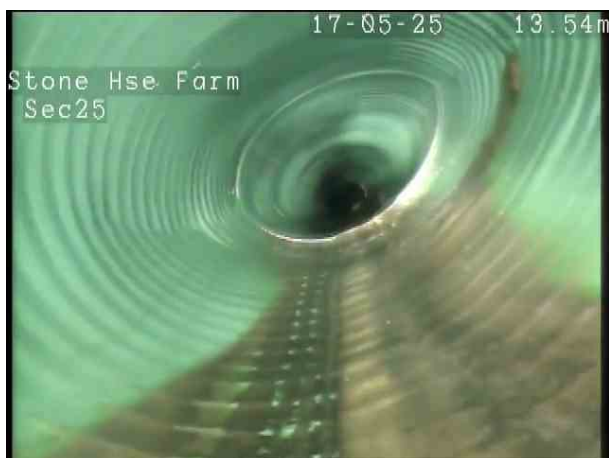
d60aa9fc-1468-4f79-8c78-2b986f9a0466.png, 00:01:56, 15.00 m Deformed sewer or drain, 40%
