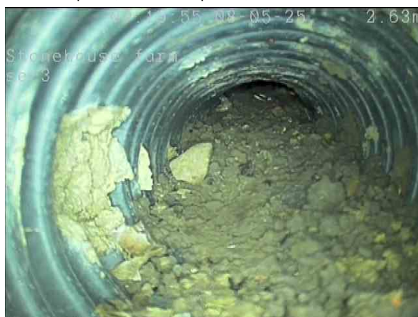
4a59a6f4-f902-4ad8-a4dc-1fd9c0eb0ec5.png, 00:00:34, 2.60 m Survey abandoned, debris obstruction
