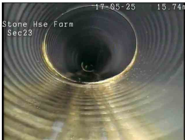
4973f8fa-a4dd-46b9-a7fa-4798b6d62da2.png, 00:01:42, 15.80 m Deformed sewer or drain, 15%
