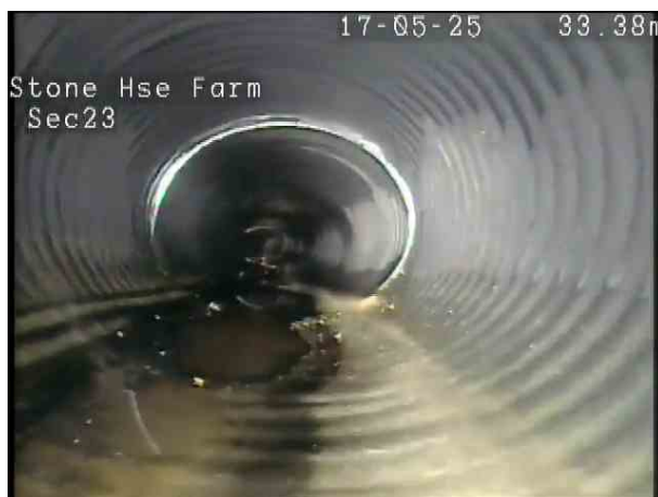
20de7bb8-8fe2-4148-8d71-5c2c8eef8bbf.png, 00:03:03, 33.50 m Deformed sewer or drain, 30%
