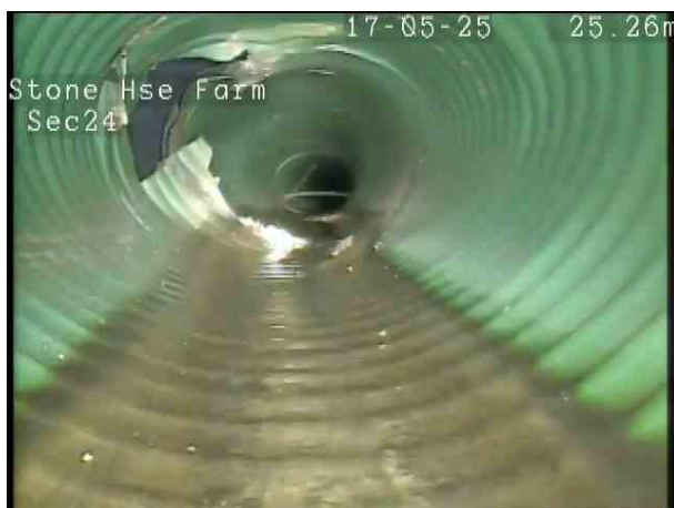
8723efe1-6fb0-46fb-851b-dca3ea5e6a30.png, 00:03:26, 25.50 m Hole in drain or sewer from 6 o'clock to 1 o'clock
