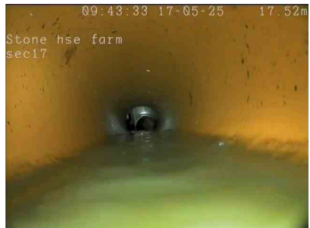
3f39e37d-07b3-444a-928f-b10e31b89f1d.png, 00:01:41, 17.50 m Water level, 10% of the vertical dimension
