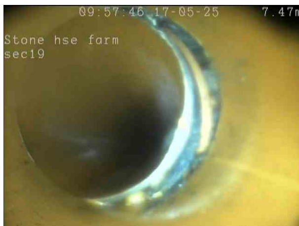
6a75b795-7754-47b7-8ad7-7f96e83b2660.png, 00:00:23, 7.50 m Joint displaced, large
