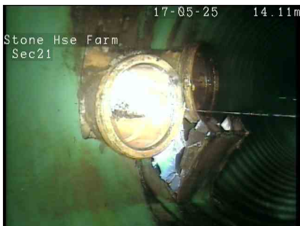
9b915c5f-7883-4957-8e8a-63928149a281.png, 00:02:10, 14.10 m General photograph taken at this point, intruding connections
