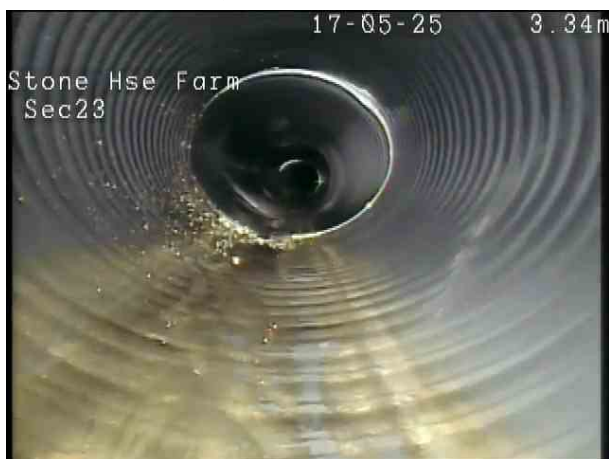
a291e06e-86b9-4d0a-8080-ff11faed5702.png, 00:00:26, 3.50 m Deformed sewer or drain, 20%
