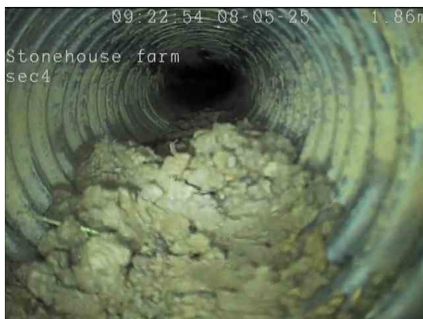
dca98030-e1be-4a14-a5d0-54d0d1180ac0.png, 00:01:19, 2.00 m Settled deposits, fine, 30% cross-sectional area loss
