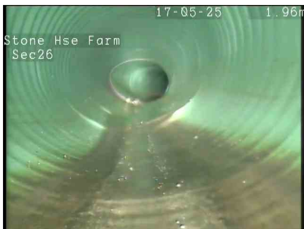
99be0dd0-8085-4999-af15-a050bc3b126f.png, 00:00:19, 2.00 m Deformed sewer or drain, 15%
