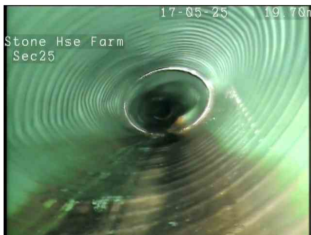
4b5bf9e6-0468-462a-862a-3b1cce96eed4.png, 00:02:42, 20.00 m Deformed sewer or drain, 35%
