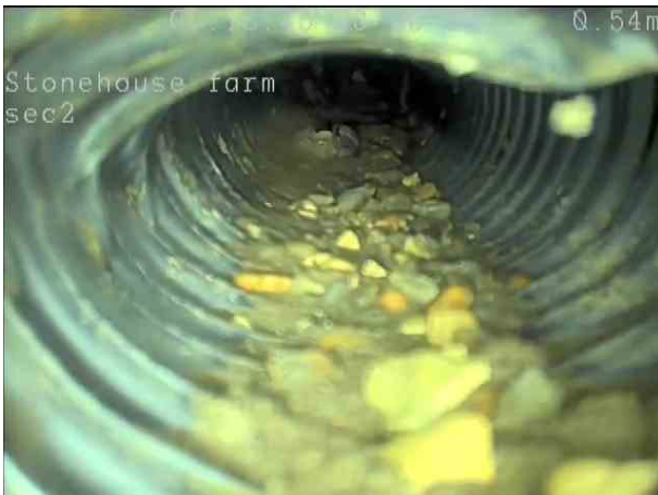
7f5fed46-c9d2-4481-a70f-404c7437758f.png, 00:00:28, 0.50 m Survey abandoned, crushed pipe work
