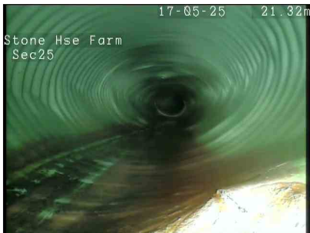
04469363-1e13-401b-948c-22050c378e6c.png, 00:03:53, 21.30 m Survey abandoned, deformed
