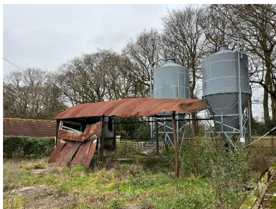
Photograph 4. B2 exterior from south.
