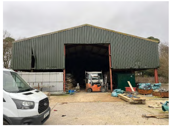
Photograph 2. B6 exterior, from the south.
