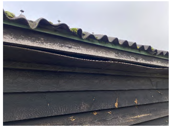
Photograph 2. Warped plywood coming away from soffit box on B6.
