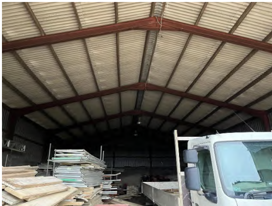
Photograph 3. B6 interior, from the south
