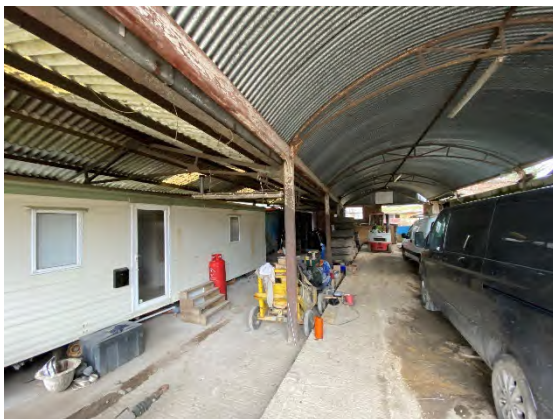
Photograph 5. Interior of B3.
