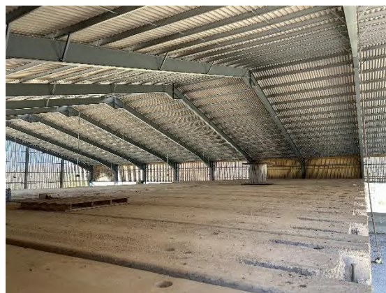
Photograph 2. The mezzanine space present within B1.
