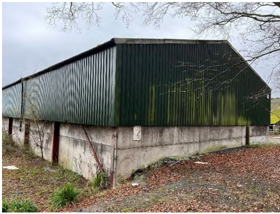
Photograph 1. B6 exterior, from the north-east.
