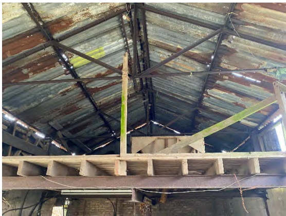
Photograph 5. Interior of B4 and inaccessible first floor
