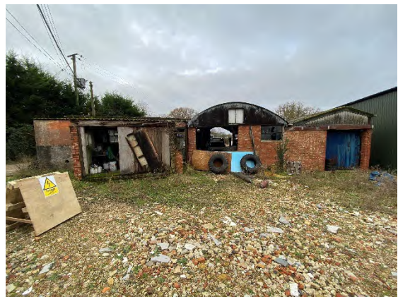
Photograph 4. Southern aspect of B3.
