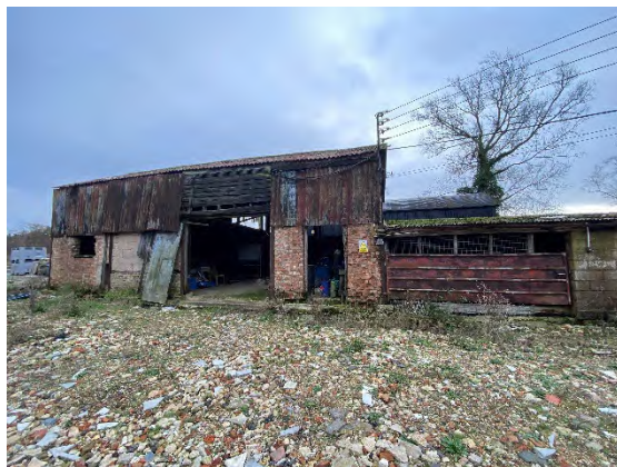
Photograph 4. B4 viewed from the north
