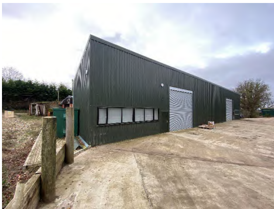
Photograph 3. B2 exterior from east. No internal access.
