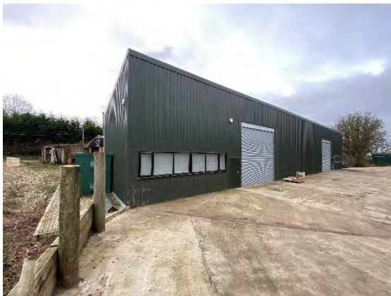
Photograph 3. B2 exterior from east. No internal access.
