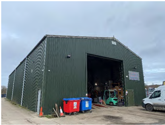
Photograph 1. B1 external from south.
