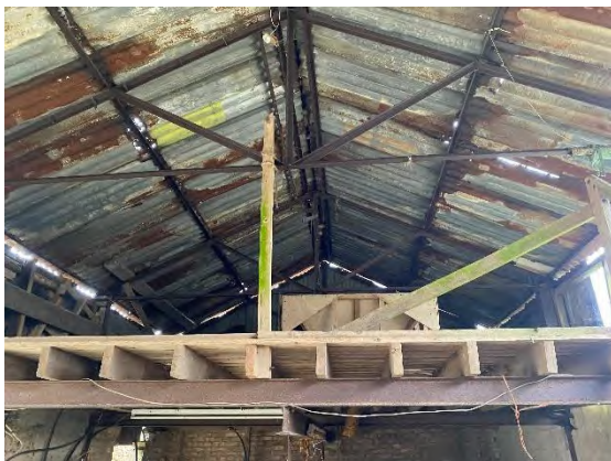
Photograph 5. Interior of B4 and inaccessible first floor
