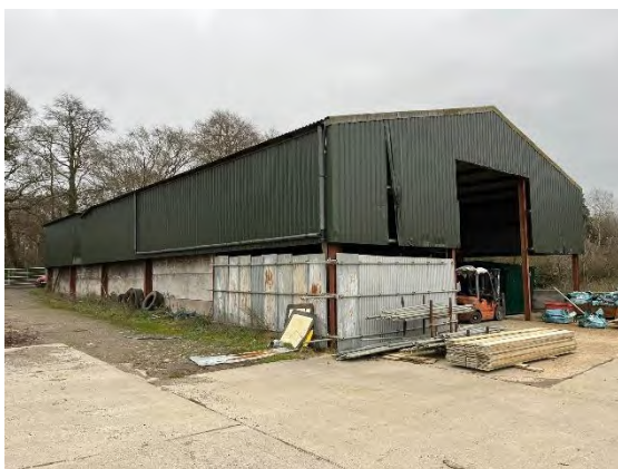
Photograph 1. Jackson's Ridge- Building B6.
