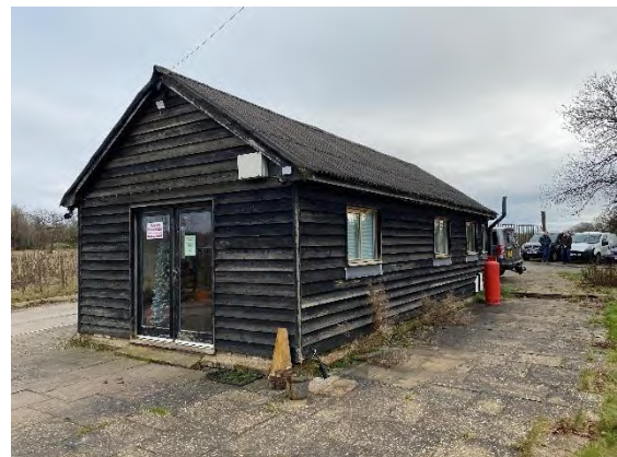
Photograph 6. Building B6 viewed from the north.
