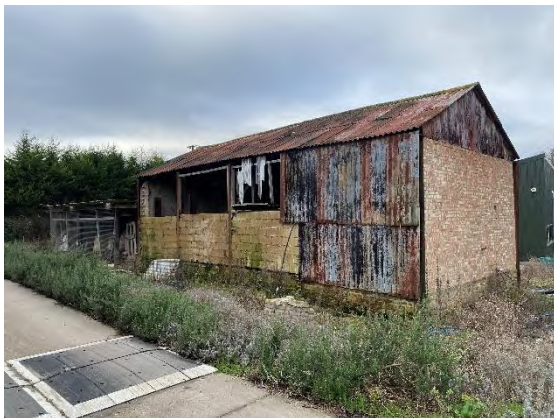
Photograph 3. B4 viewed from the south
