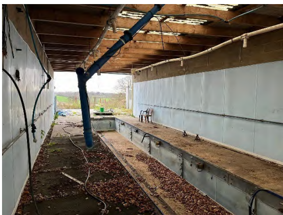
Photograph 7. Interior wall of B4, open to south.
