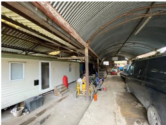
Photograph 5. Interior of B3.
