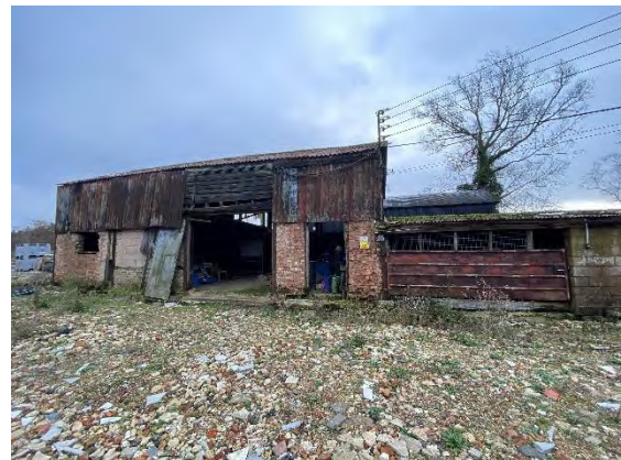
Photograph 4. B4 viewed from the north
