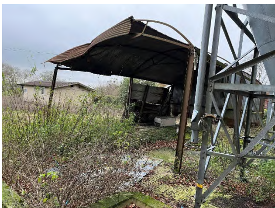
Photograph 3. B2 exterior from north-east.
