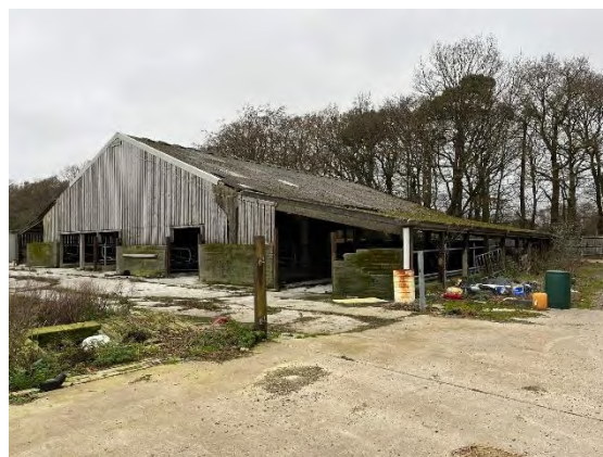
Photograph 2. Jackson's Ridge- Building B5.
