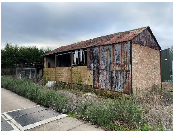
Photograph 3. B4 viewed from the south
