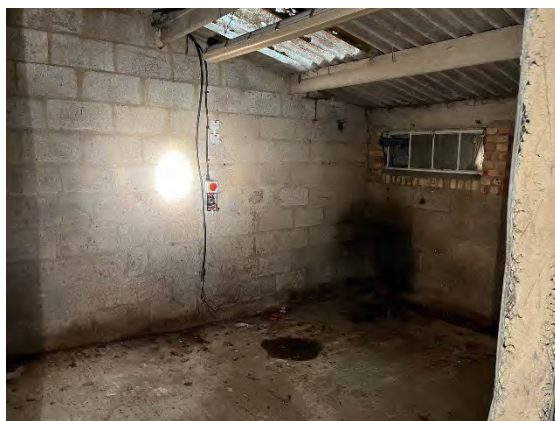
Photograph 12. B5 interior (ground floor, north)
