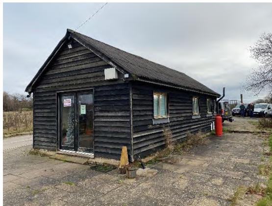
Photograph 6. Building B6 viewed from the north.
