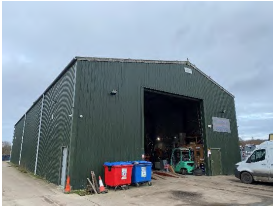
Photograph 1. B1 external from south.
