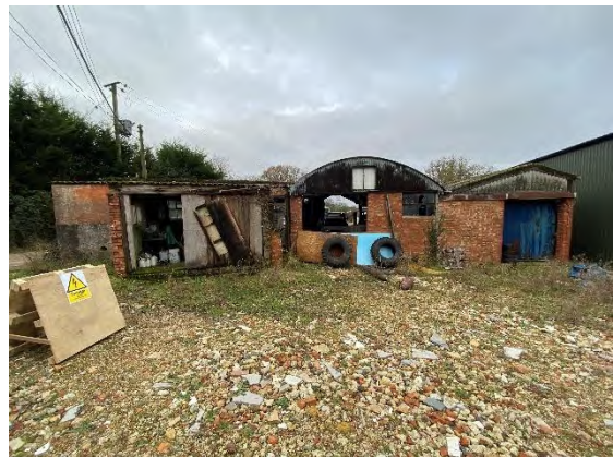
Photograph 4. Southern aspect of B3.
