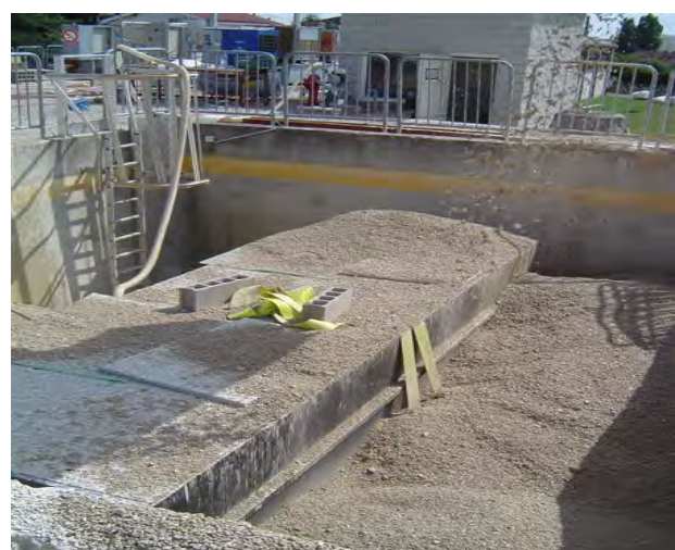
Backfilling with gravel to include the maximum backfill authorised and the pedestrian loads
