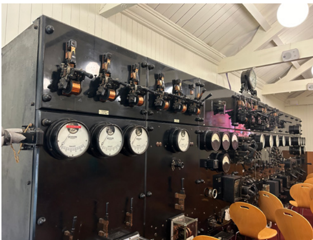
The control panel for monitoring the generators and their supply within the powerhouse at Waddesdon Manor
