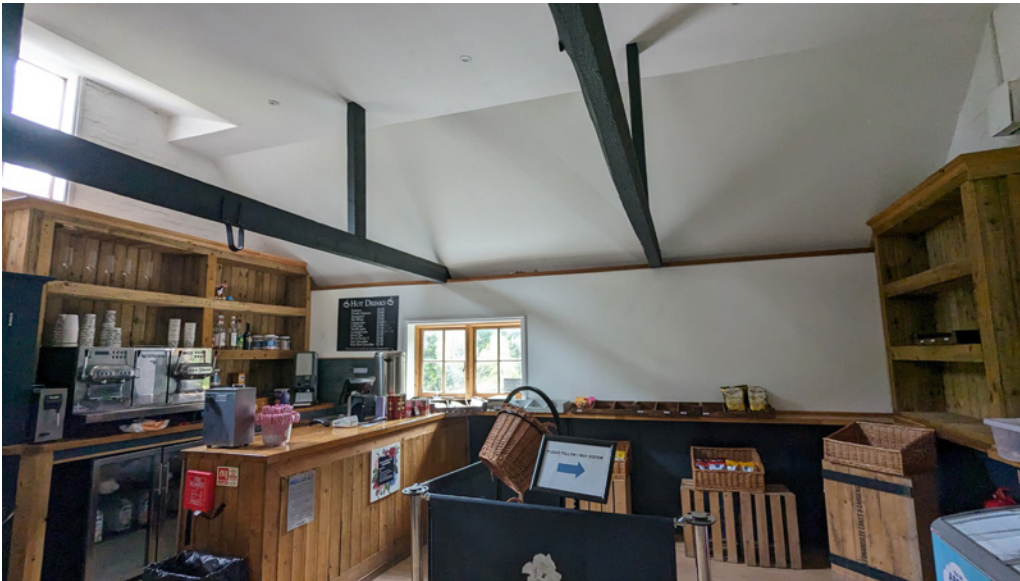
Engine House interior featuring exposed tie beams
