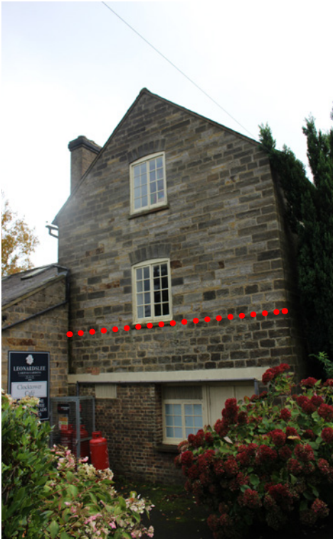
North elevation of west range showing a disparity in stonework between the lower and upper levels as shown by the red dotted line. The image also shows the ground floor brick facing, reflecting the presence of a former structure that was later removed.
