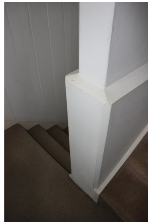
Historic stair newel post with chamfered edges
