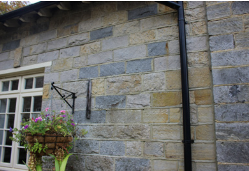
Vertical joint between the main part of the east range and Honey Cottage
