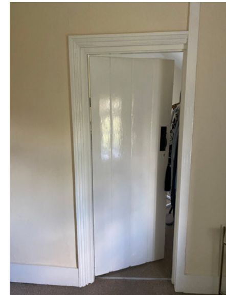
Historic boarded door at first-floor level (modern architrave)
