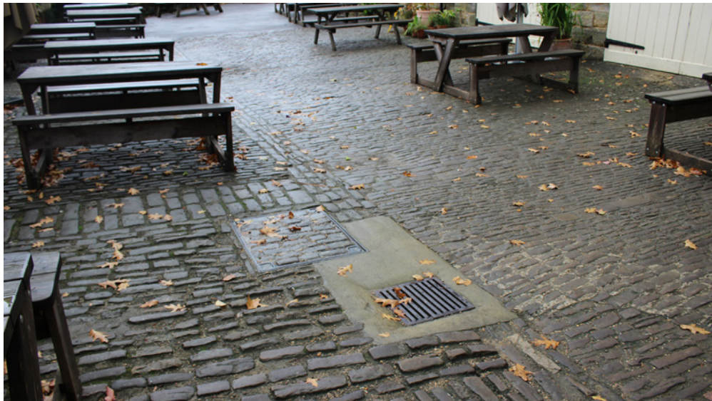
Cobbles within the stable yard showing areas of modern alteration
