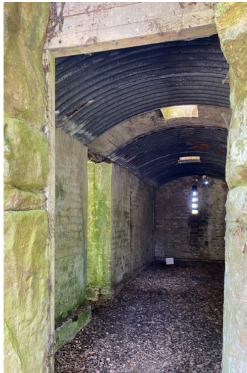
View of the interior of the rockwork showing structural brick walls and corrugated metal ceiling cladding
