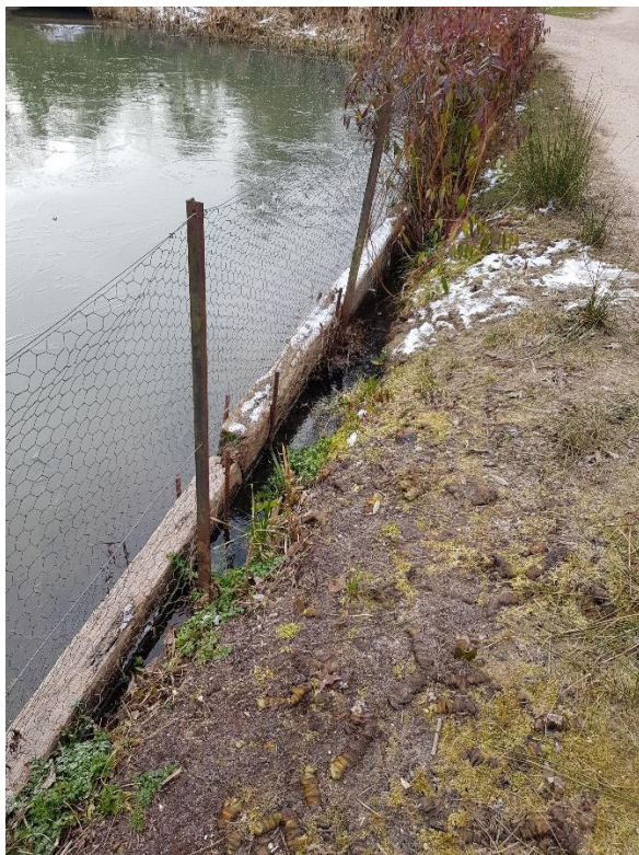
5. Examples of path/lake edge erosion and undercutting
