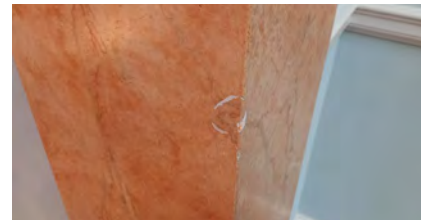
Plate 6.41 - Example of damage to the paintwork on the pilasters
