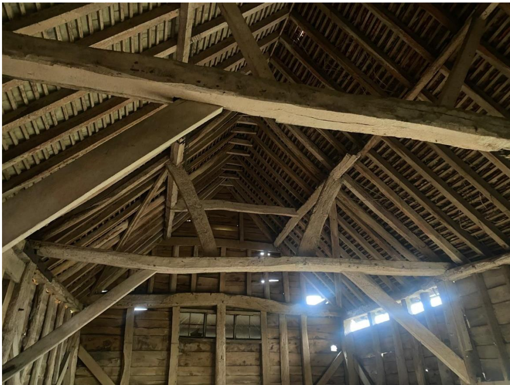
Photo 8 – Internal view of tiled roof without membrane.
