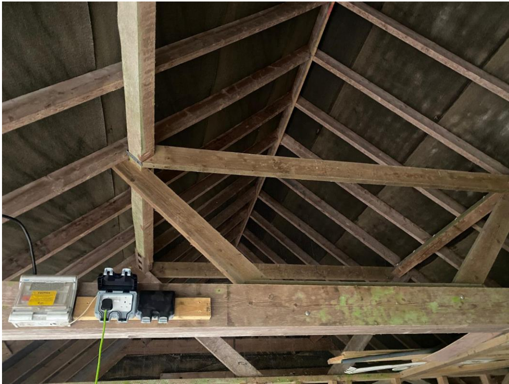
Photo 7 – Internal view of wooden rafters and internal membrane.
