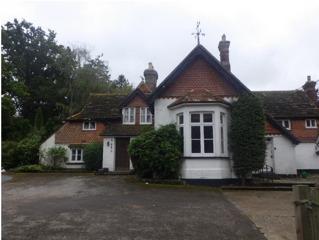
Plate 14: Front view of house
