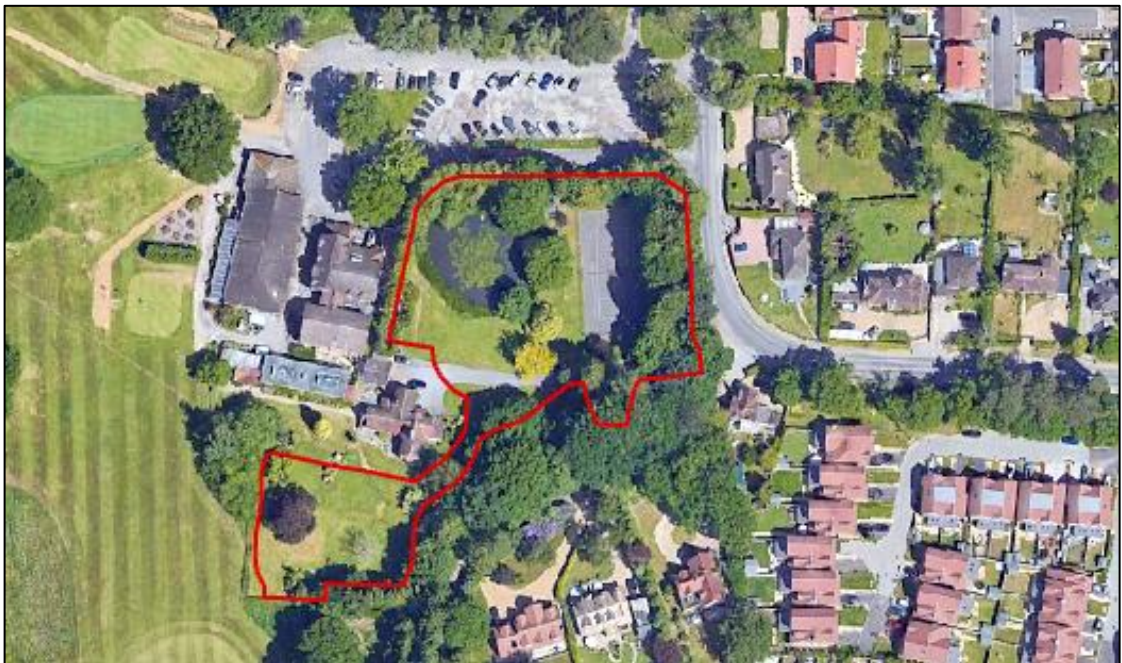
Aerial View 2025 (Goggle Earth Pro)
