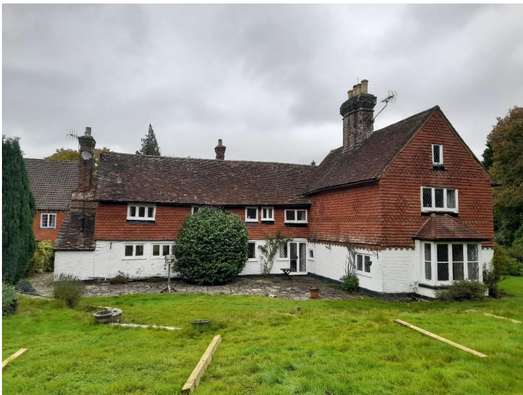
Plate 16: House from south-west
