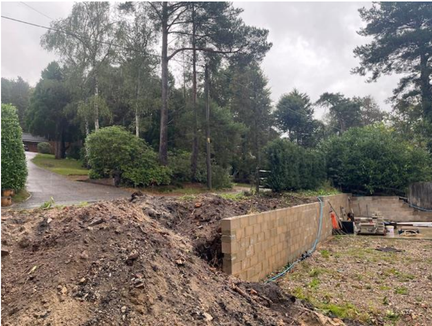
New retaining wall and groundworks adjacent to Bracken Lane, Storrington
