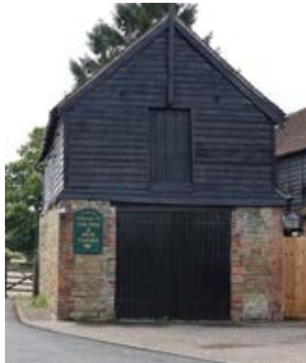
Local architectural precedents of brick and timber weather boarding with low eaves lending a humble appearance to buildings
