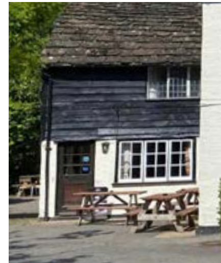
Local architectural precedents of brick and timber weather boarding with low eaves lending a humble appearance to buildings
