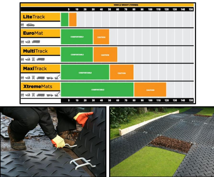
5.3.14 Ground protection is to be laid following erection of the TPF but prior to the commencement of any soil stripping, and will remain in place for the duration of the project. It will be removed immediately prior to the landscaping phase once all heavy plant has been removed from site.
