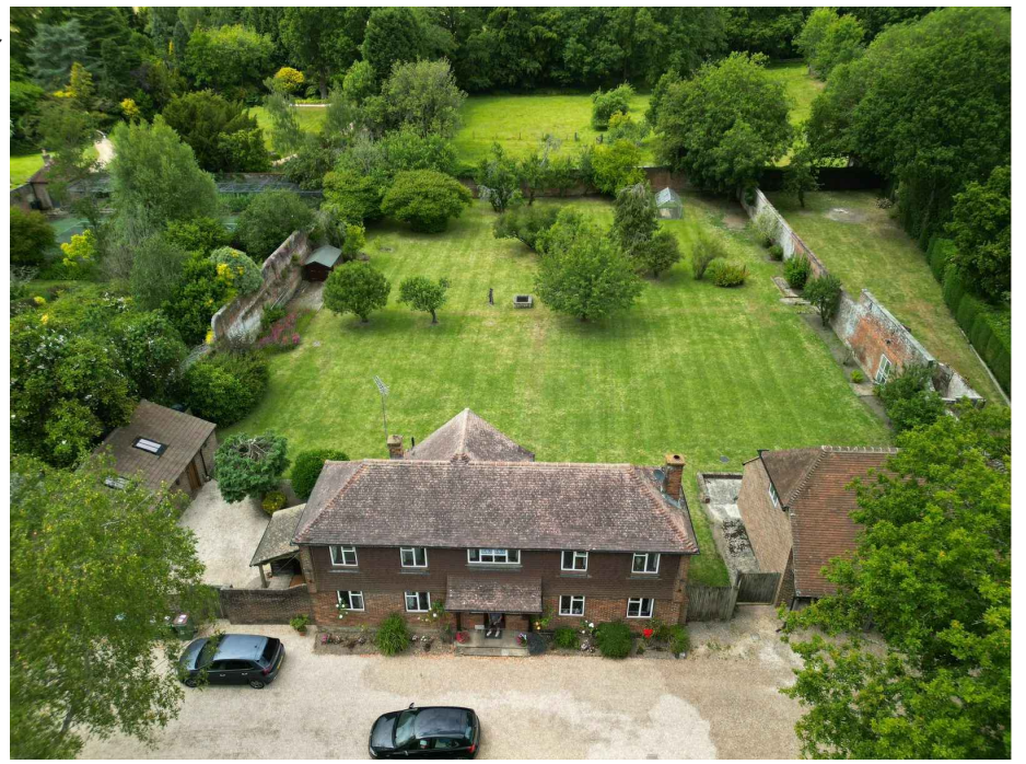
This view from the front shows how the high garden walls will conceal the proposed extension from view. This view also shows where the link between the existing house and garage will not project past the existing front elevation. The existing porch can also be seen, the proposed new porch not projecting past the line of the existing steps.
