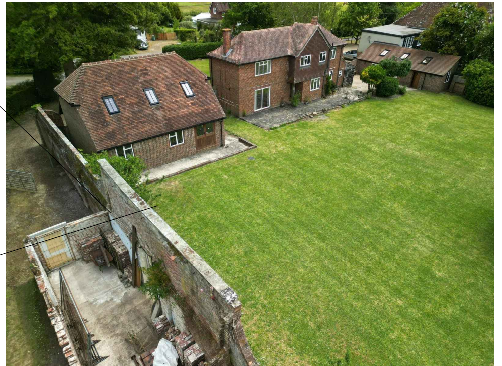
View of the rear elevation showing the height of the garden wall ( not on the boundary) and how this wall obscures the view of the proposed extension for the neighbouring properties.
