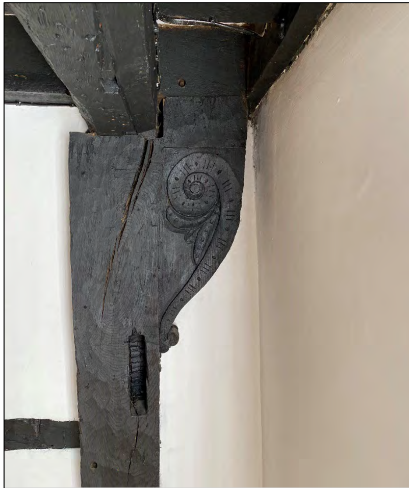
Figure 1: Evidence of carved jetty in the first floor front bedroom, showing later extension to right
