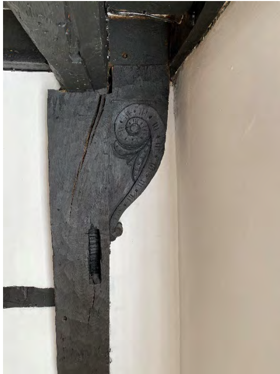
Figure 25 – First Floor Front Jetty Detail South
