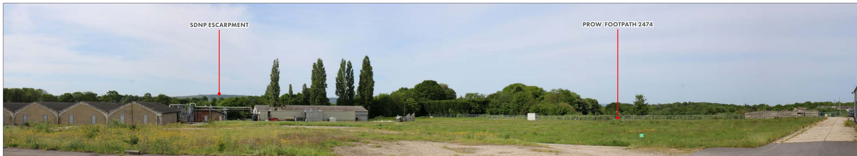
UPDATED PHOTOGRAPH – VIEWPOINT E VIEW LOOKING SOUTH FROM THE CENTRE OF THE SITE. THE EXISTING BUILDINGS, SOUTHERN BOUNDARY VEGETATION (WITH POPLAR TREES) AND HARD STANDING IS APPARENT. SECURITY FENCING AND DISUSED CRATES FORM DETRACTING FEATURES. THE SDNP ESCARPMENT IS VISIBLE IN THE DISTANT HORIZON.
