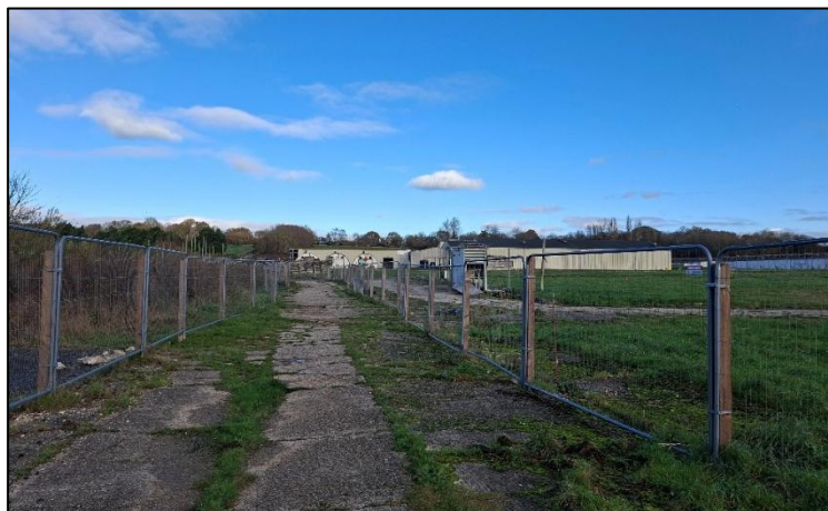
Figure 2.1: View of some of the building extant on the Site
