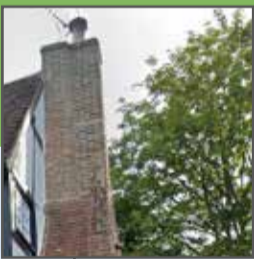
EXTERNAL CHIMNEY STACK
