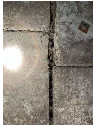
Photograph 4. B6, limited extent of expansion gaps between concrete panels on internal walls.
