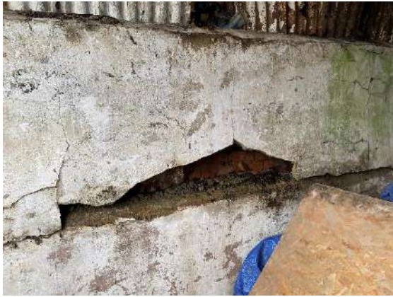
Photograph 1. Interior wall of B3 that has crumbled.
