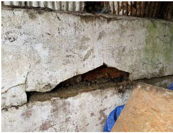
Photograph 1. Interior wall of B3 that has crumbled.
