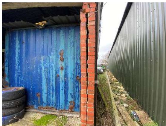
Photograph 6. External wall of B3 forming crack crevice.
