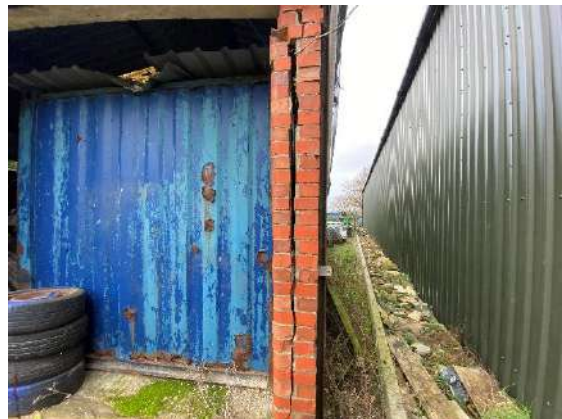
Photograph 6. External wall of B3 forming crack crevice.
