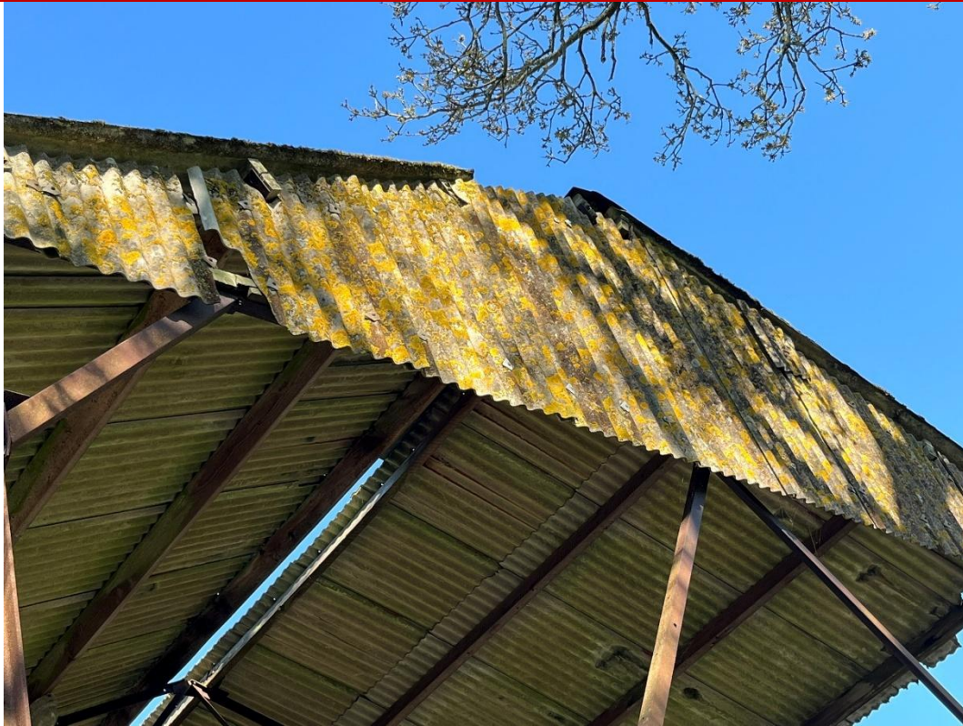
Photo 11 – Suspected asbestos cement on the western barn with fragments missing.
