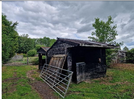
Stable 1 (Structure 5)- Wooden clad design with felt roofing over corrugated concrete sheets.
