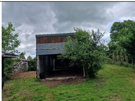
Hay barn (Structure 6) with open front entrance. Tin roof and part tin and wooden clad design.
