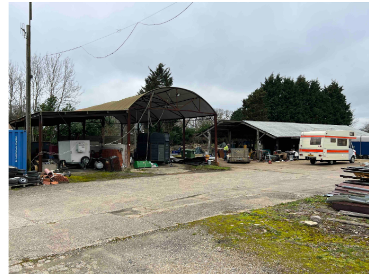
Figure 2.2 - Existing Open Barns To Be Demolished
