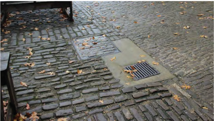
Cobbles within the stable yard showing areas of modern repair and alteration
