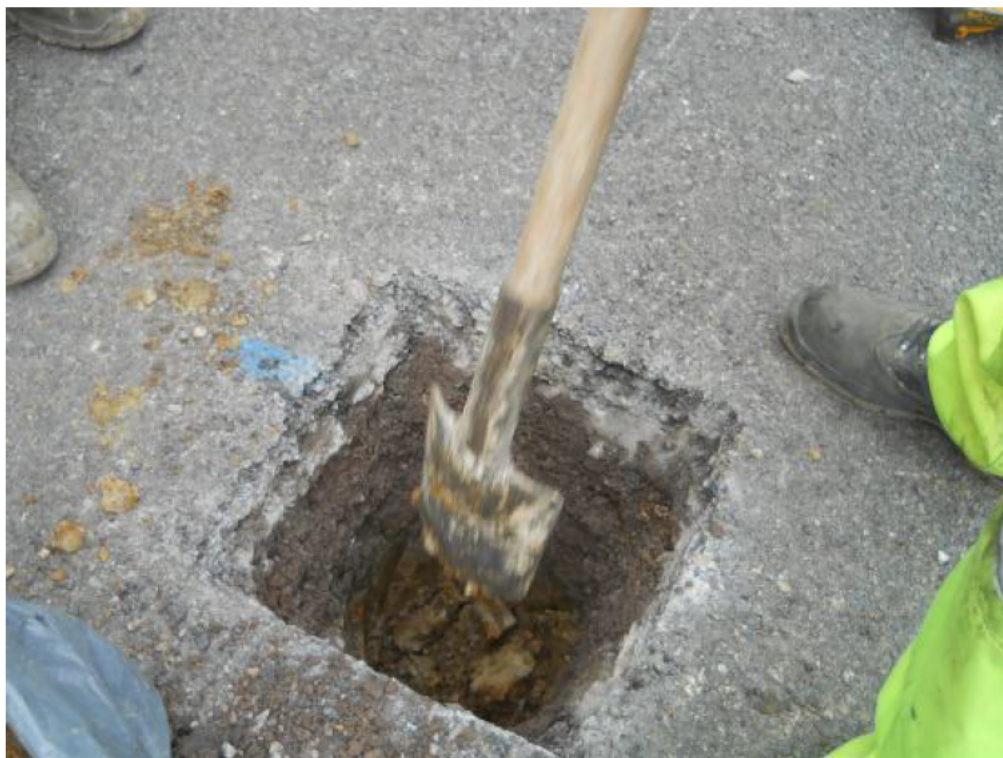
WS56 – hand digging through made ground
