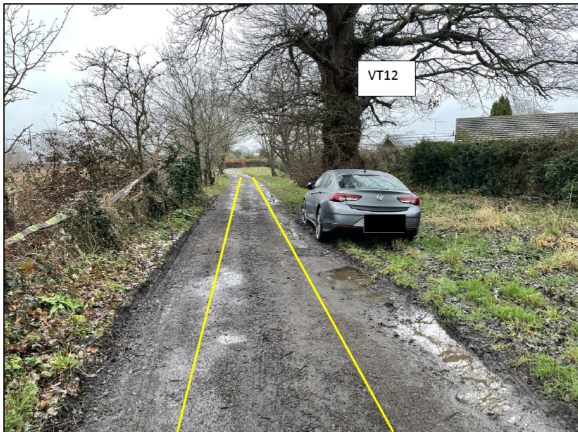
Photo 1: Looking south along the existing access track. The existing tarmac surface will be carefully removed and a new footpath (no vehicular access) will be installed approximately where the yellow are shown which will be narrower than the existing track and constructed using a cellular confinement system improving the available rooting zone for the trees adjacent to the access, including VT1 & VT12.
