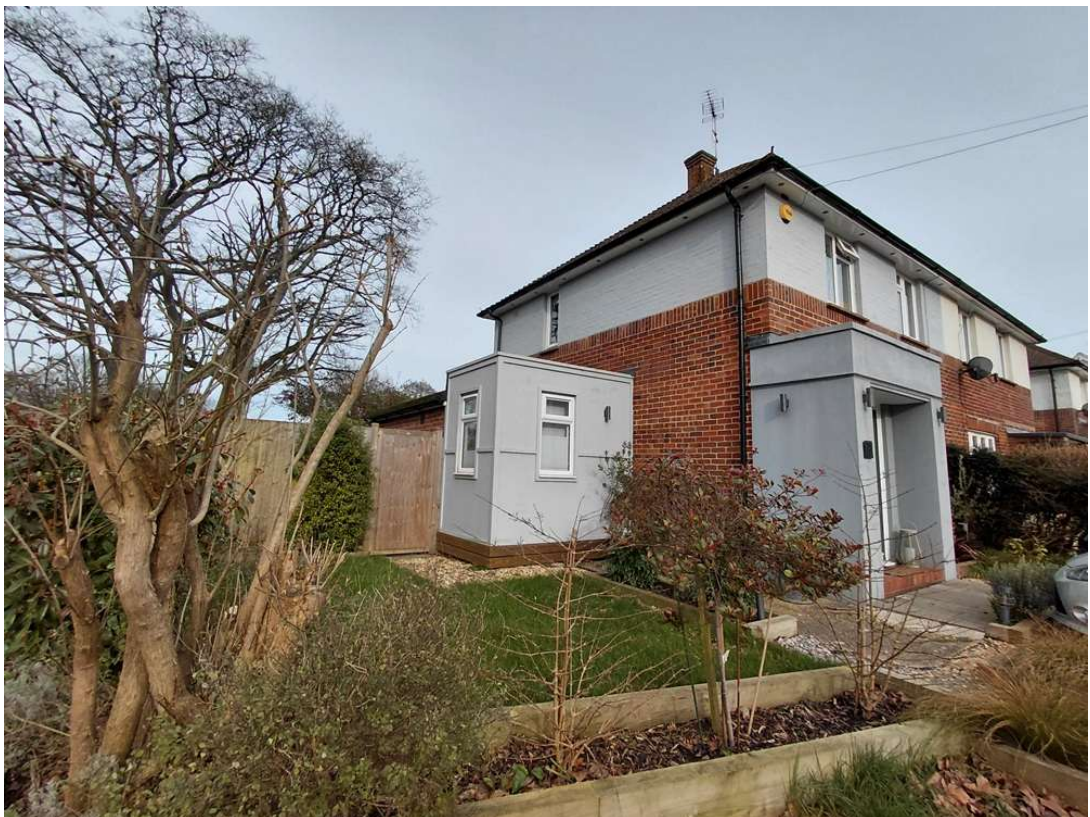
Front-side of Subject Site- No. 25 - Above
