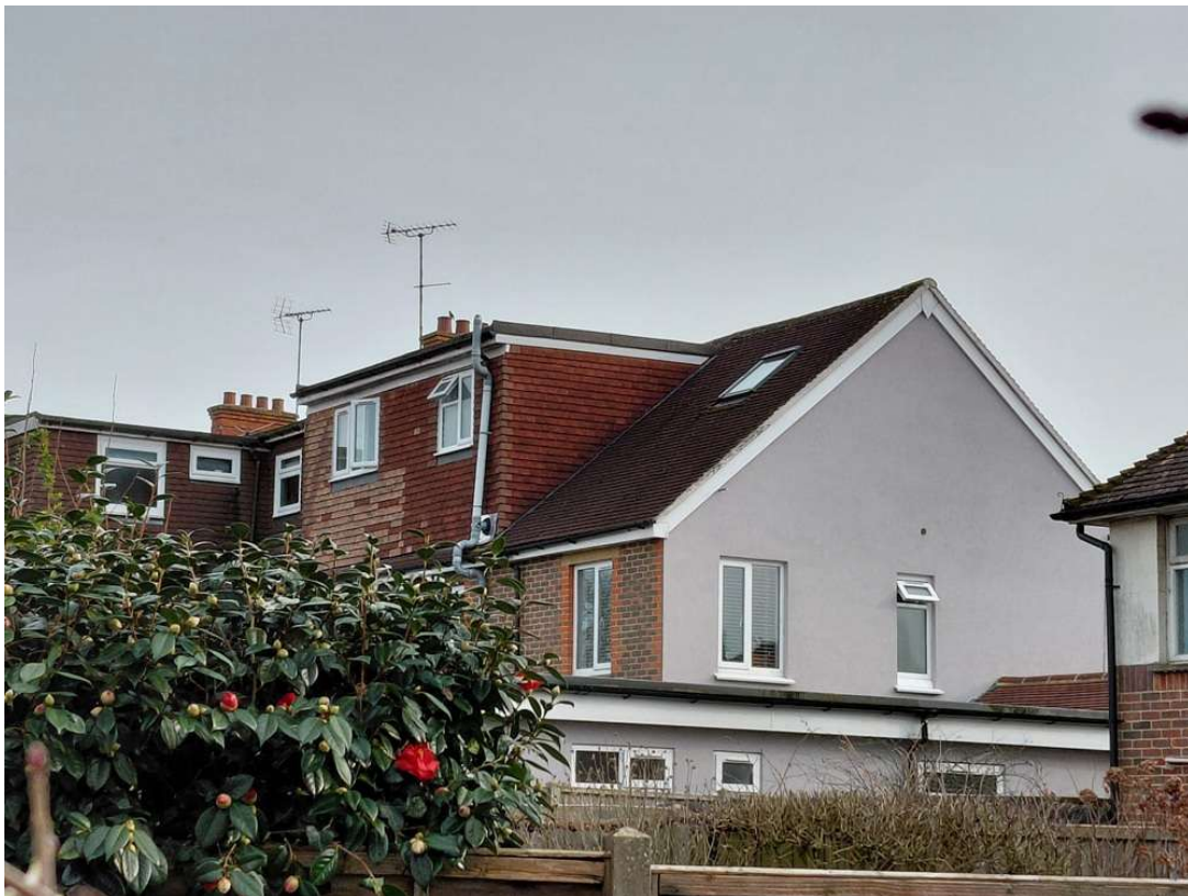
Neighbouring Properties of Subject Site- No. 25- Above
