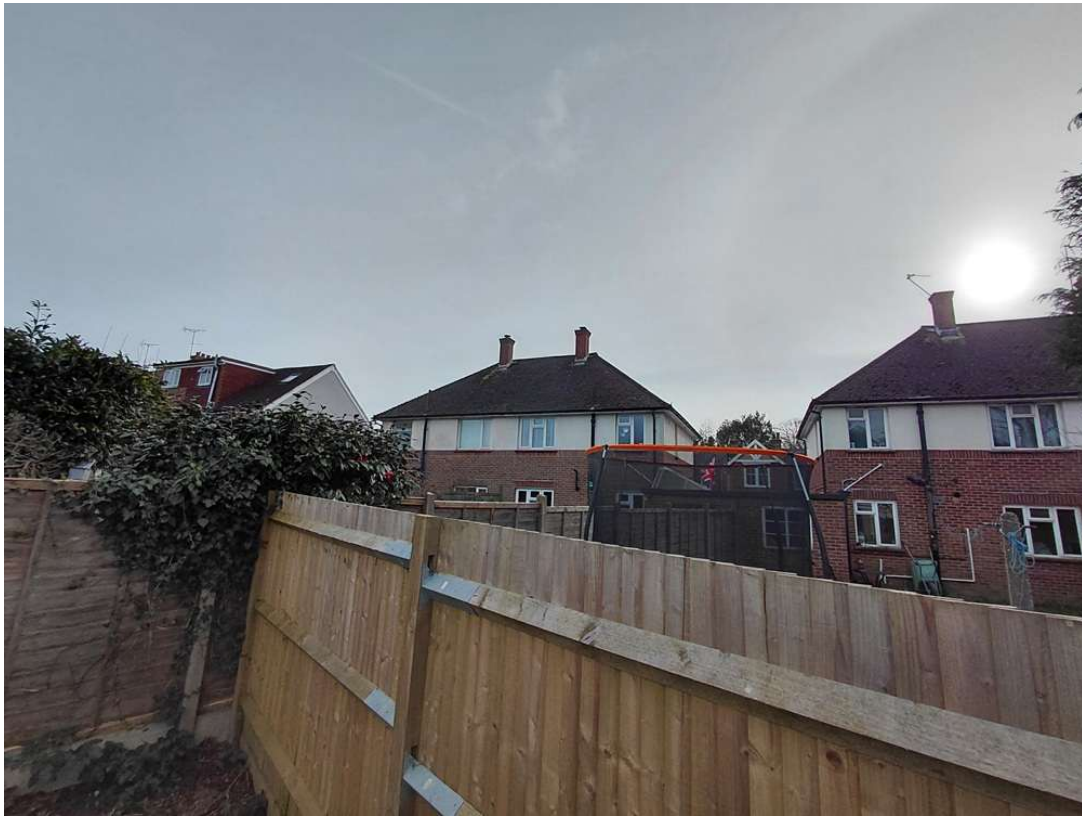
Rear of Neighbouring Properties of Subject Site- No. 25- Above
