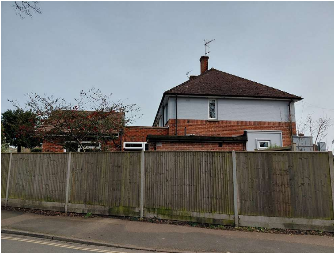
Side of Subject Site- No. 25 - Above
