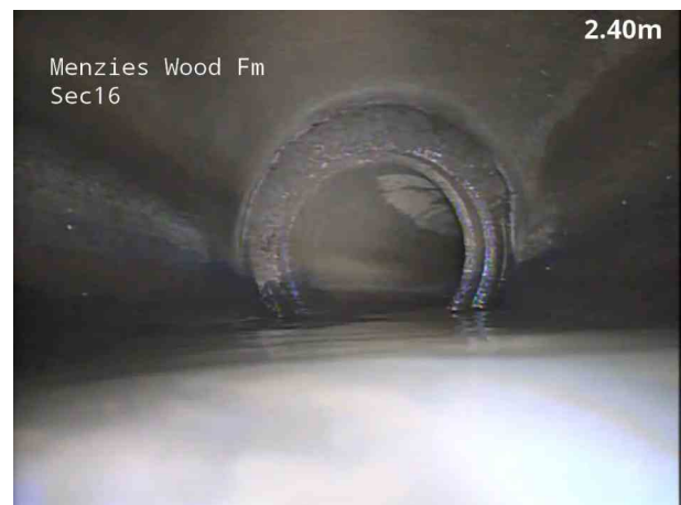
4, 00:00:35, 2.40 m Water level, 20% of the vertical dimension
