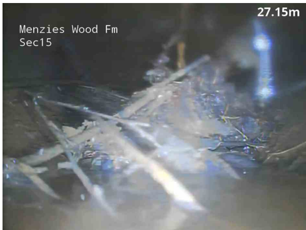
7, 00:04:00, 27.15 m Roots, mass, 25% cross-sectional area loss
