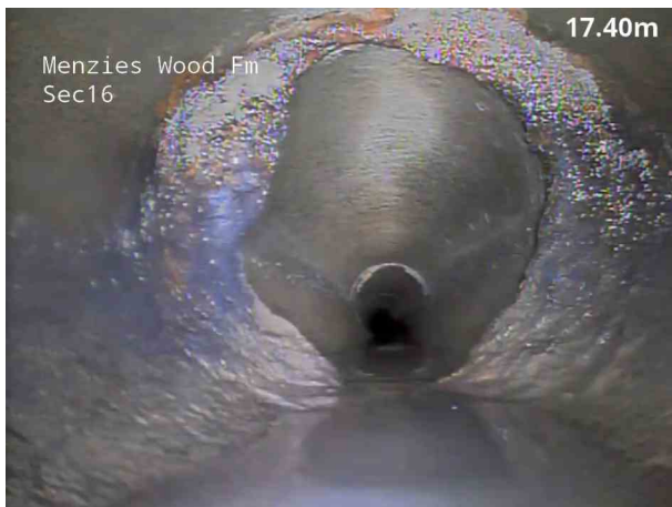
11, 00:01:55, 17.60 m Attached deposits, encrustation at joint from 12 o'clock to 12 o'clock, 40% cross-sectional area loss
