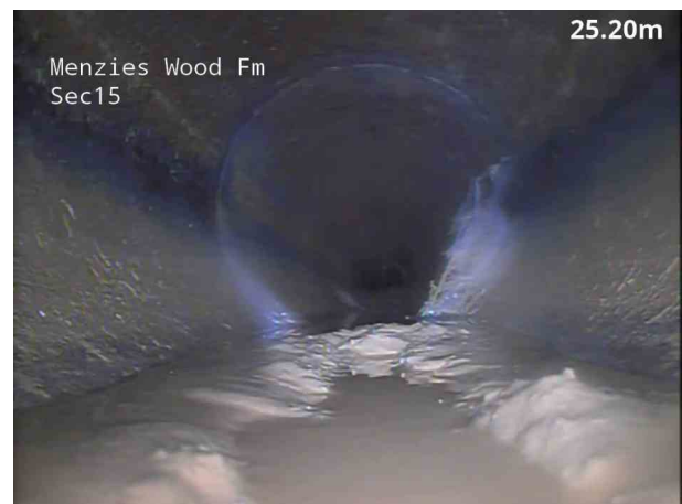
6, 00:03:31, 25.40 m Settled deposits, fine, 10% cross-sectional area loss
