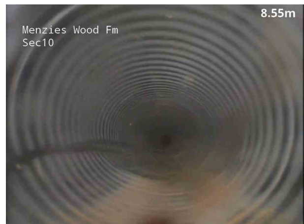
6, 00:01:19, 8.50 m Settled deposits, fine, 10% cross-sectional area loss, finish
