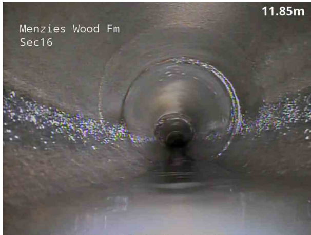
7, 00:01:19, 12.10 m Fracture, circumferential from 12 o'clock to 12 o'clock
