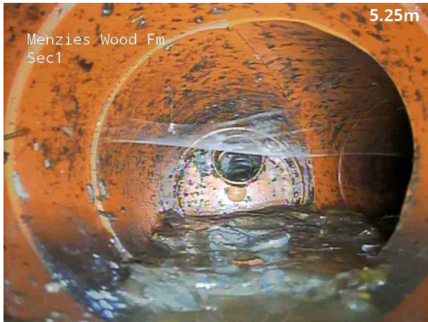
7, 00:01:18, 5.30 m Junction at 3 o'clock, 100mm dia
