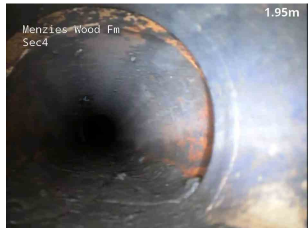
6, 00:00:46, 1.95 m Joint displaced, medium
