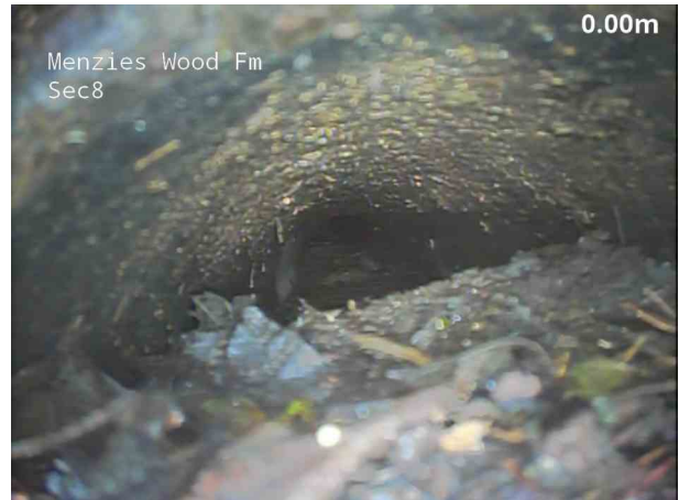
2, 00:00:04, 0.00 m Settled deposits, coarse, 85% cross-sectional area loss, start
