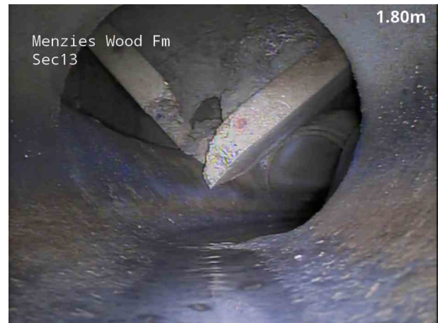
2, 00:00:21, 2.10 m Finish node, manhole, reference: SW7, Buried. Cover collapsed
