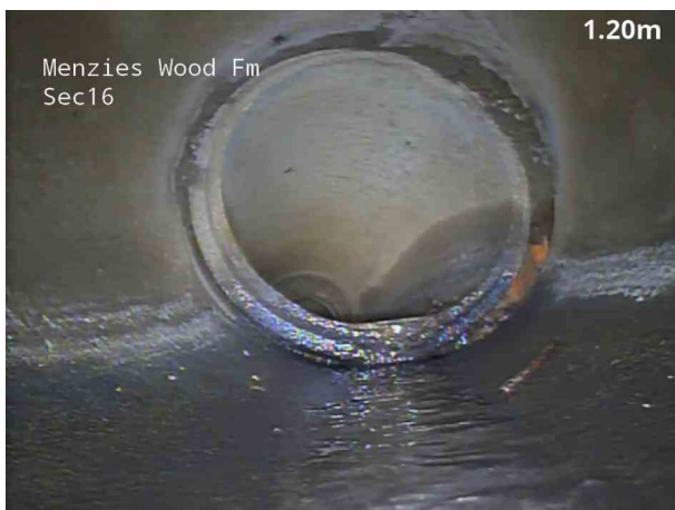
3, 00:00:18, 1.40 m Pipe size changes, new size(s), 225mm high, 225mm wide
