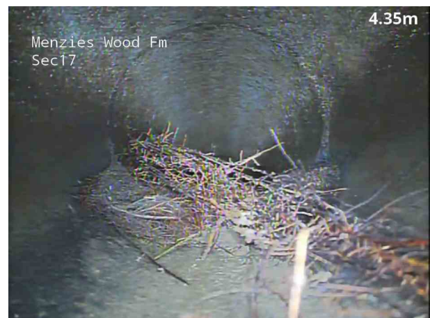
4, 00:00:31, 4.50 m Roots, mass at joint, 15% cross-sectional area loss
