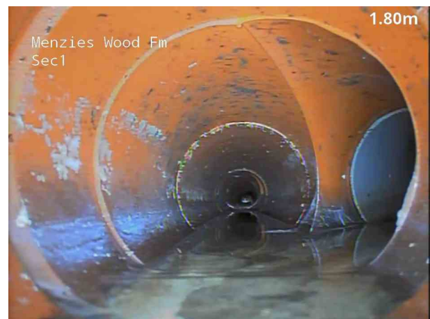
4, 00:00:36, 2.00 m Junction at 3 o'clock, 100mm dia
