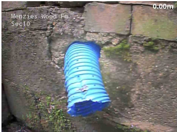
1, 00:00:00, 0.00 m Start node, catchpit, reference: SW4, Perforated land drain
