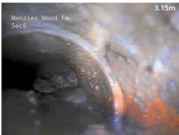
5, 00:00:51, 3.60 m Settled deposits, coarse, 100% cross-sectional area loss
