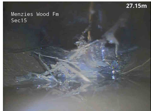
8, 00:03:55, 27.40 m Roots, mass at joint, 40% cross-sectional area loss
