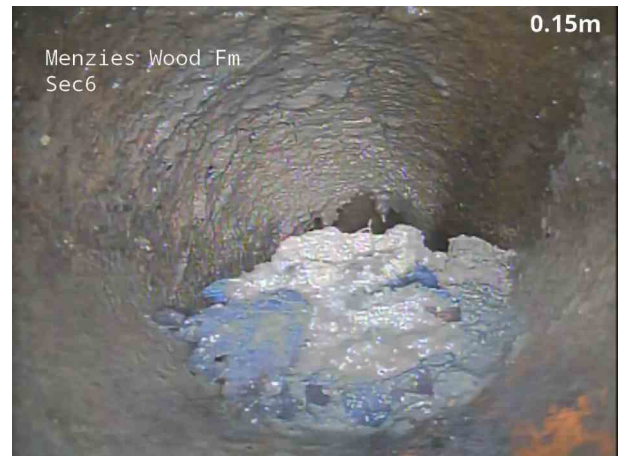
2, 00:00:06, 0.30 m Settled deposits, fine, 50% cross-sectional area loss
