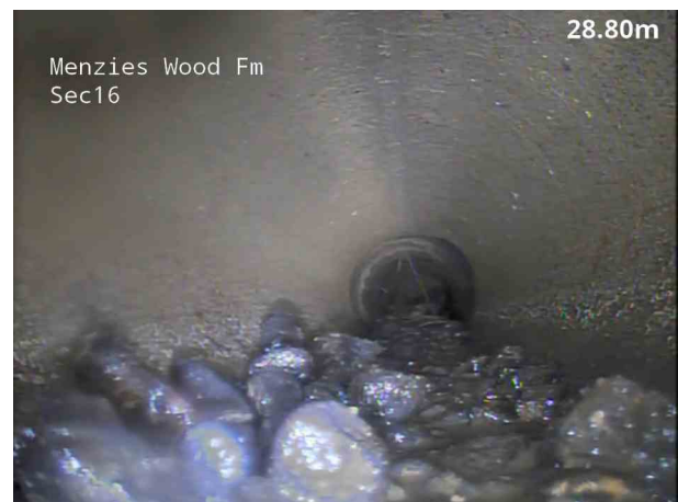
16, 00:02:55, 28.80 m Settled deposits, coarse, 15% cross-sectional area loss, start
