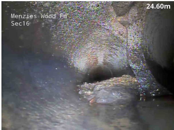
13, 00:02:26, 24.90 m Settled deposits, hard or compacted, 20% cross-sectional area loss, start
