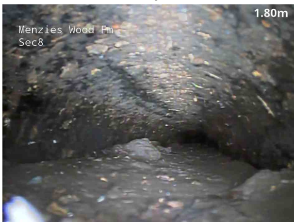
5, 00:00:44, 2.00 m Settled deposits, coarse, 70% cross-sectional area loss, change
