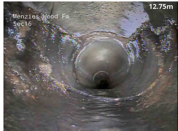
10, 00:01:33, 12.80 m Fracture, circumferential from 3 o'clock to 9 o'clock
