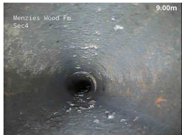
10, 00:02:03, 9.00 m Settled deposits, hard or compacted, 10% cross-sectional area loss, change
