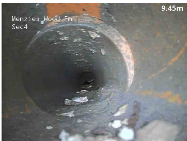
11, 00:02:07, 9.60 m Joint displaced, medium
