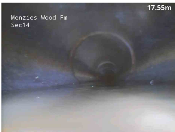
3, 00:00:50, 17.50 m Water level, 10% of the vertical dimension
