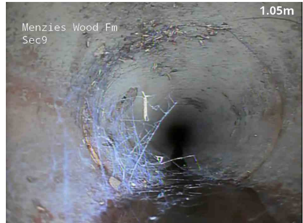
2, 00:00:14, 1.20 m Fracture, circumferential from 12 o'clock to 12 o'clock
