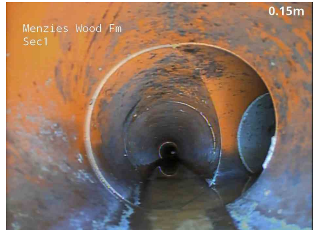
2, 00:00:15, 0.30 m Junction at 3 o'clock, 100mm dia
