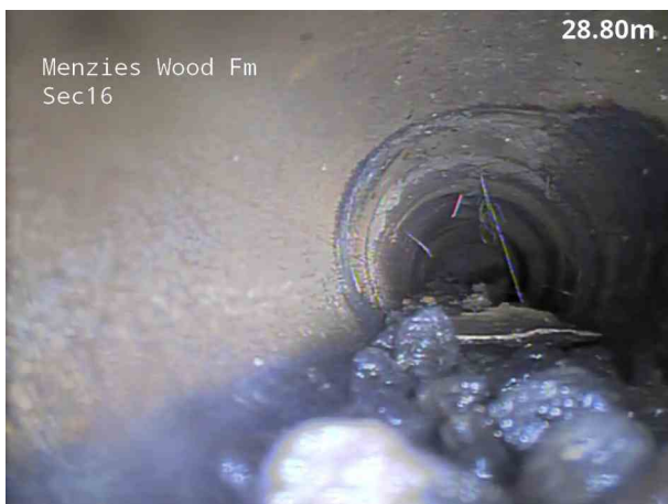
17, 00:03:04, 29.00 m Settled deposits, coarse, 25% cross-sectional area loss, change
