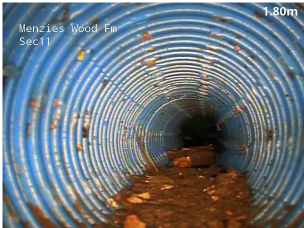
3, 00:00:28, 2.00 m Settled deposits, fine, 15% cross-sectional area loss, start
