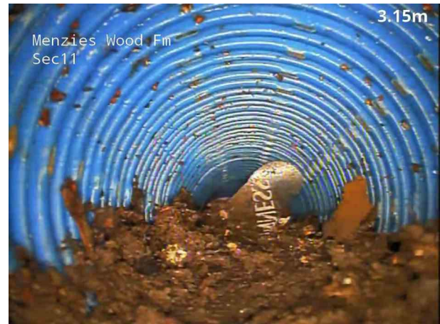
4, 00:00:50, 3.20 m Settled deposits, fine, 50% cross-sectional area loss, change
