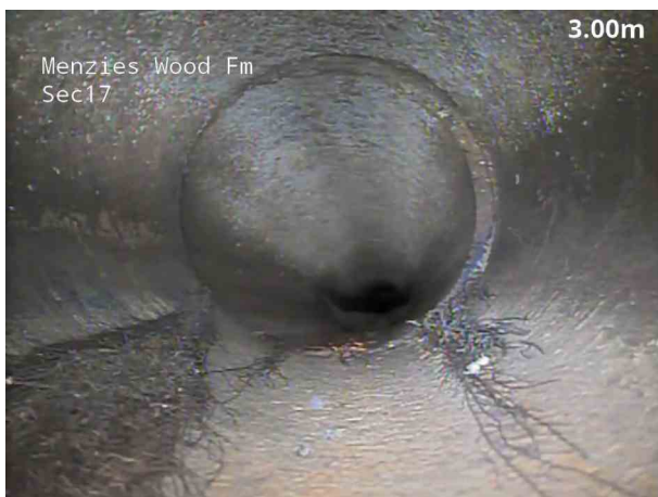
3, 00:00:20, 3.30 m Roots, fine at joint
