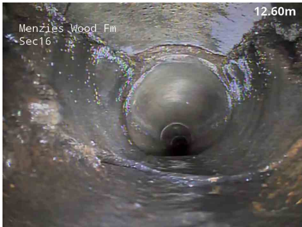
9, 00:01:26, 12.70 m Point repair, hole repaired from 10 o'clock to 2 o'clock
