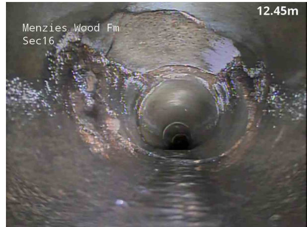
8, 00:01:26, 12.70 m Point repair, hole repaired from 10 o'clock to 2 o'clock
