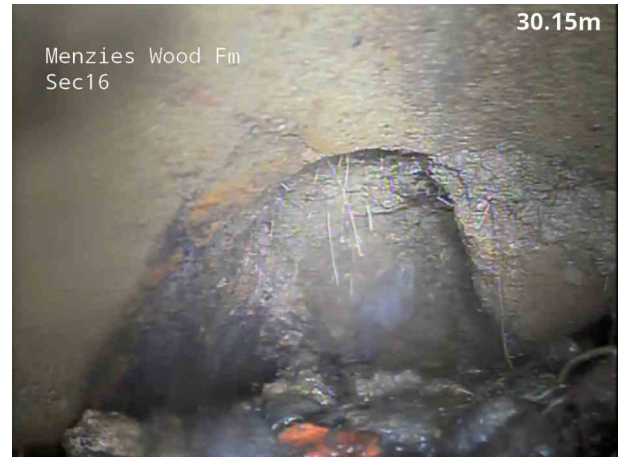
20, 00:03:26, 30.30 m Collapsed drain or sewer, 100% cross-sectional area loss
