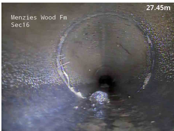
15, 00:02:48, 27.60 m Roots, fine at joint
