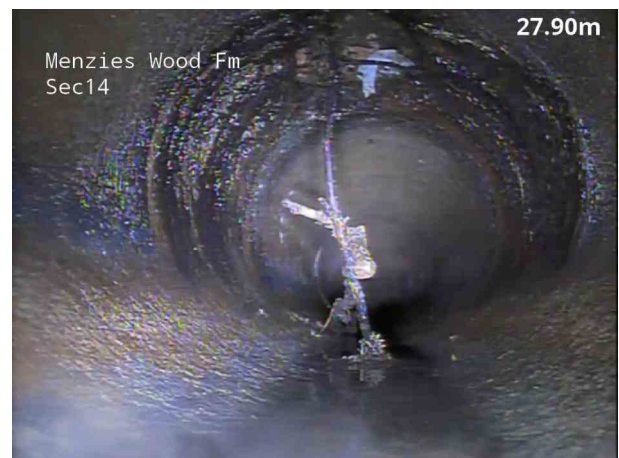
4, 00:02:02, 28.20 m Hole in drain or sewer at 12 o'clock
