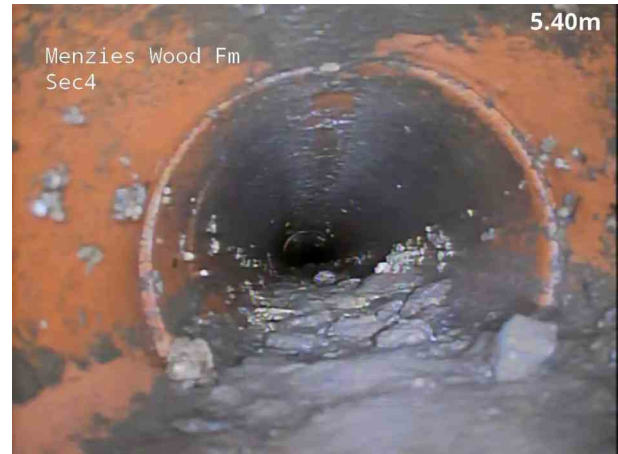
8, 00:01:30, 5.50 m Settled deposits, hard or compacted, 20% cross-sectional area loss, change
