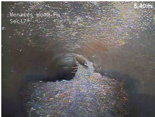
9, 00:01:15, 8.60 m Roots, mass, 55% cross-sectional area loss
