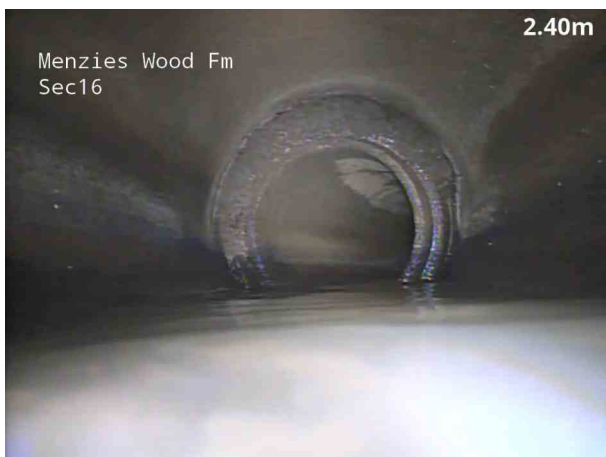
5, 00:00:35, 2.90 m Pipe size changes, new size(s), 150mm high
