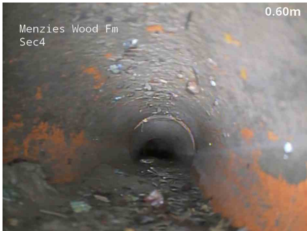
3, 00:00:31, 0.60 m Settled deposits, hard or compacted, 15% cross-sectional area loss, start
