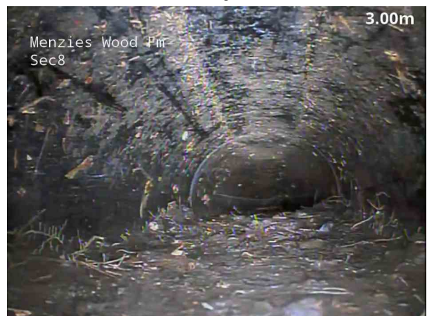
6, 00:01:10, 3.00 m Settled deposits, coarse, 60% cross-sectional area loss, change
