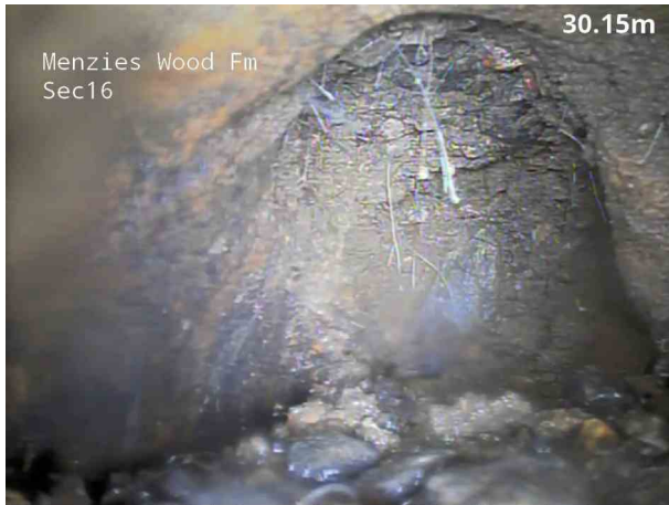
19, 00:03:26, 30.30 m Collapsed drain or sewer, 100% cross-sectional area loss
