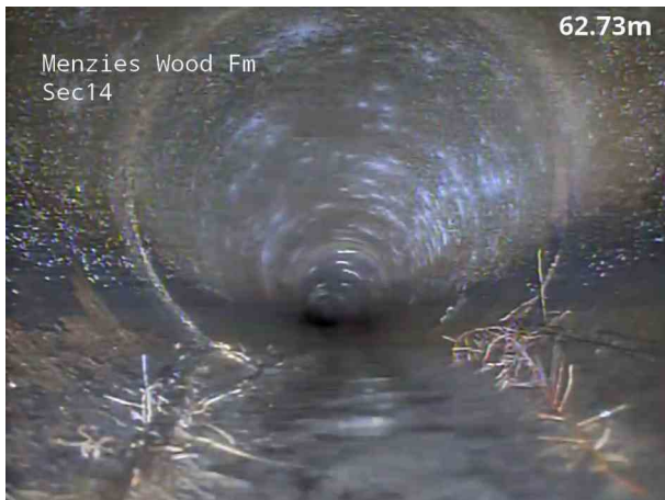
7, 00:03:28, 63.00 m Roots, fine at joint
