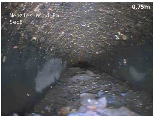
3, 00:00:23, 0.70 m Settled deposits, coarse, 45% cross-sectional area loss, change
