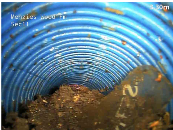
5, 00:01:24, 3.50 m Settled deposits, coarse, 90% cross-sectional area loss
