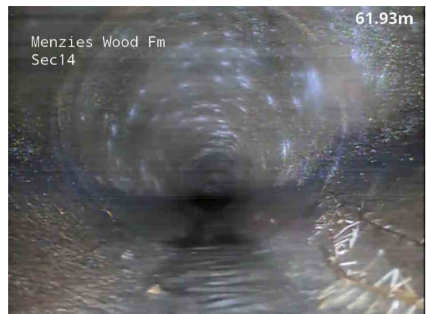
6, 00:03:23, 62.20 m Roots, fine at joint
