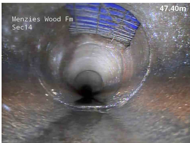
5, 00:02:53, 47.70 m Point repair, hole repaired from 11 o'clock to 2 o'clock
