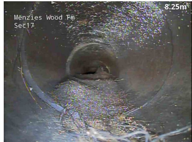
8, 00:01:05, 8.40 m Roots, mass, 20% cross-sectional area loss
