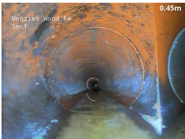
3, 00:00:22, 0.50 m Water level, 10% of the vertical dimension, Continuous
