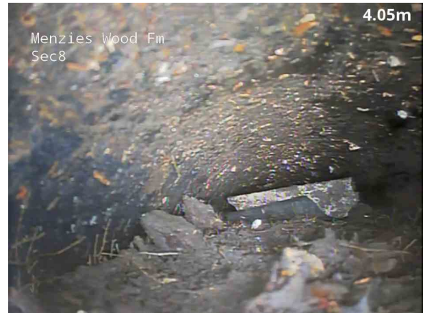
8, 00:01:29, 4.30 m Settled deposits, coarse, 90% cross-sectional area loss
