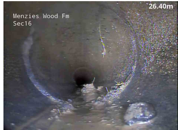
14, 00:02:42, 26.60 m Roots, fine at joint
