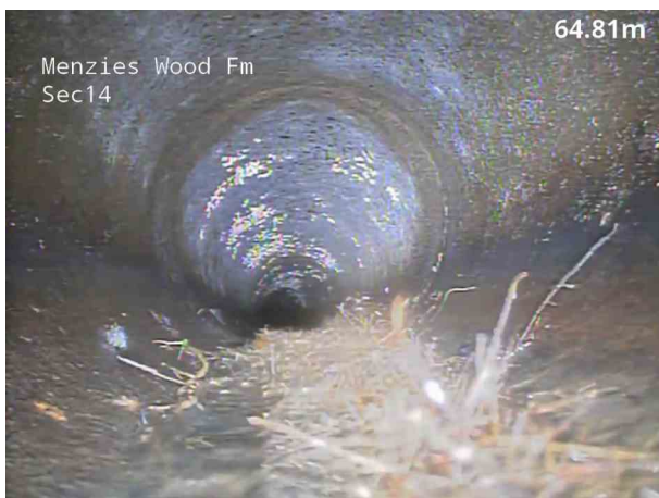
9, 00:03:55, 65.20 m Roots, mass at joint, 10% cross-sectional area loss
