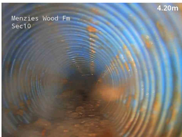
5, 00:00:52, 4.30 m Settled deposits, fine, 10% cross-sectional area loss, start
