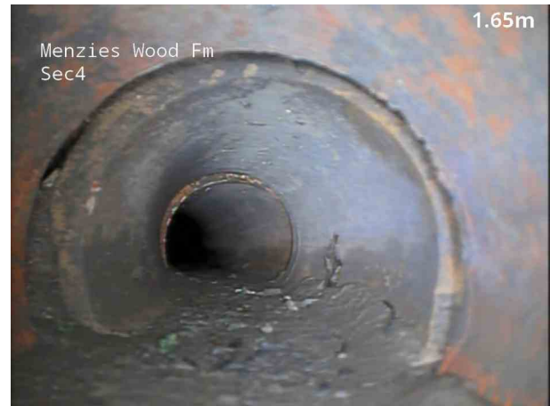
4, 00:00:39, 1.65 m Open joint, medium, open
