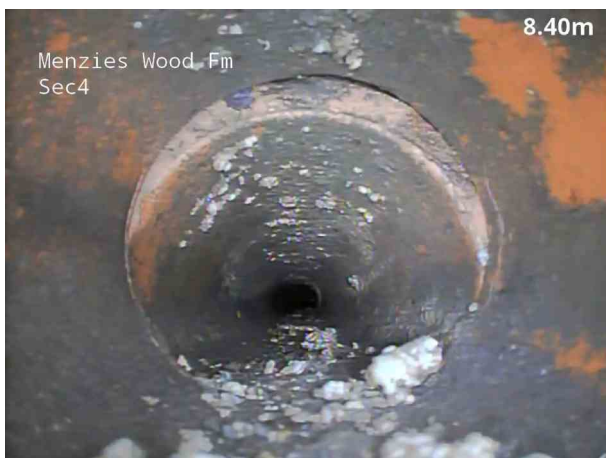
9, 00:01:56, 8.40 m Joint displaced, medium
