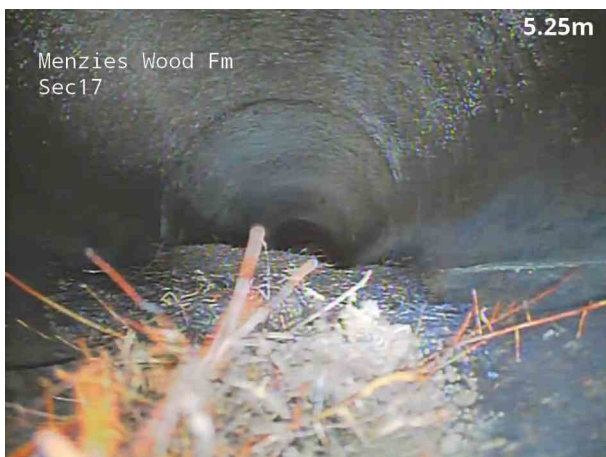
5, 00:00:44, 5.50 m Roots, mass at joint, 25% cross-sectional area loss
