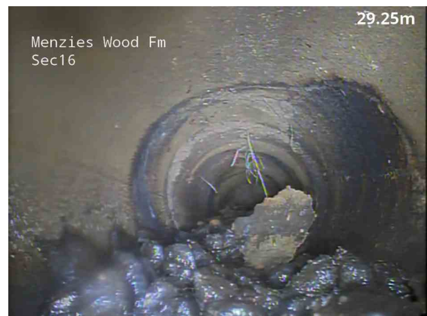
18, 00:03:08, 29.40 m Fracture, circumferential from 8 o'clock to 4 o'clock
