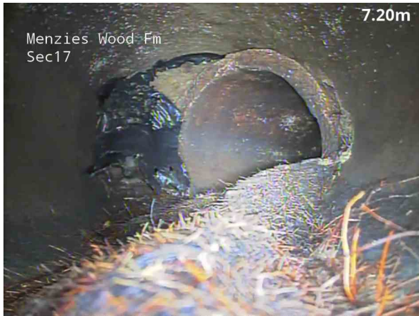
7, 00:00:56, 7.40 m Roots, mass at joint, 20% cross-sectional area loss
