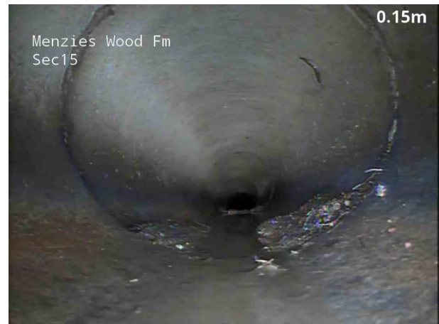
2, 00:00:07, 0.60 m Roots, fine at joint, start
