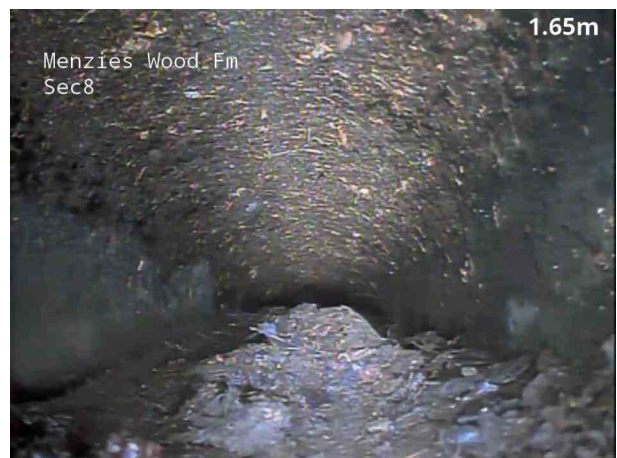
4, 00:00:33, 1.70 m Settled deposits, coarse, 55% cross-sectional area loss, change
