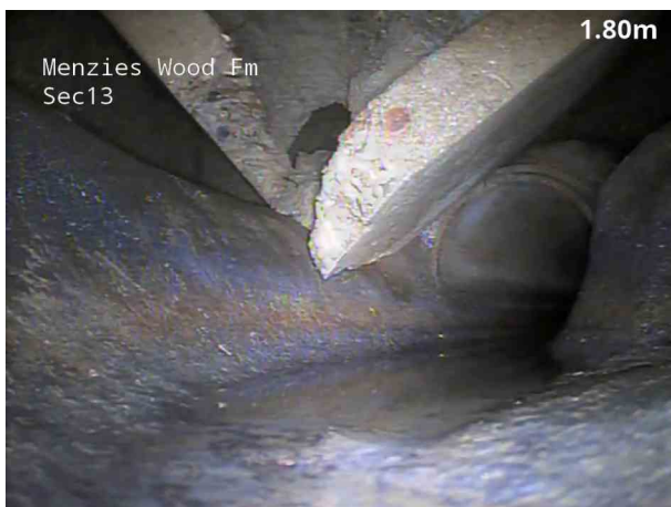
3, 00:00:21, 2.10 m Finish node, manhole, reference: SW7, Buried. Cover collapsed
