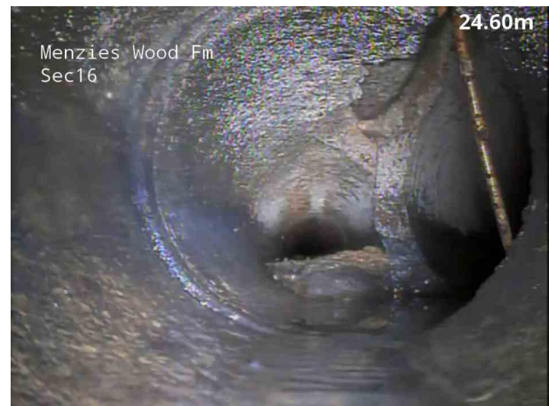
12, 00:02:23, 24.80 m Connection defective at 3 o'clock, 150mm dia, Assumed to serve neighbouring FW treatment plant
