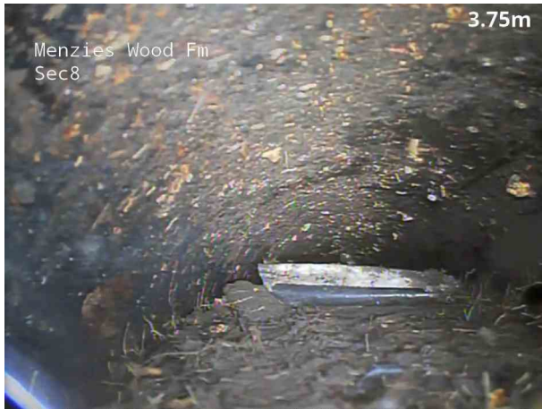
7, 00:01:21, 3.90 m Settled deposits, coarse, 80% cross-sectional area loss, change
