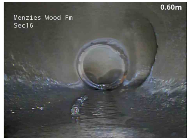
2, 00:00:13, 1.00 m Junction at 3 o'clock, 300mm dia
